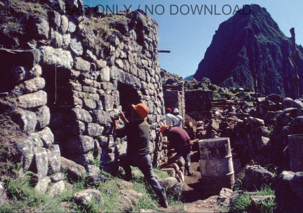
Figure E.2. Restoration work in the "Industrial Group."
