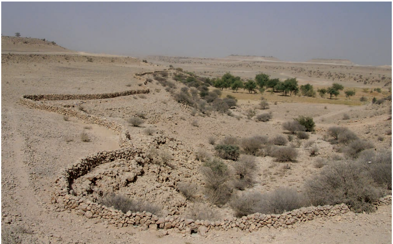
Figure 13.6. Stone wall built to slow runoff and prevent erosion above Wadi Do'an. Photograph by Michael Harrower.
