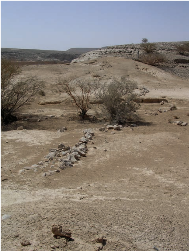
Figure 13.3. Check dam in small tributary drainage along Wādī Sanā. Photograph by Michael Harrower.
