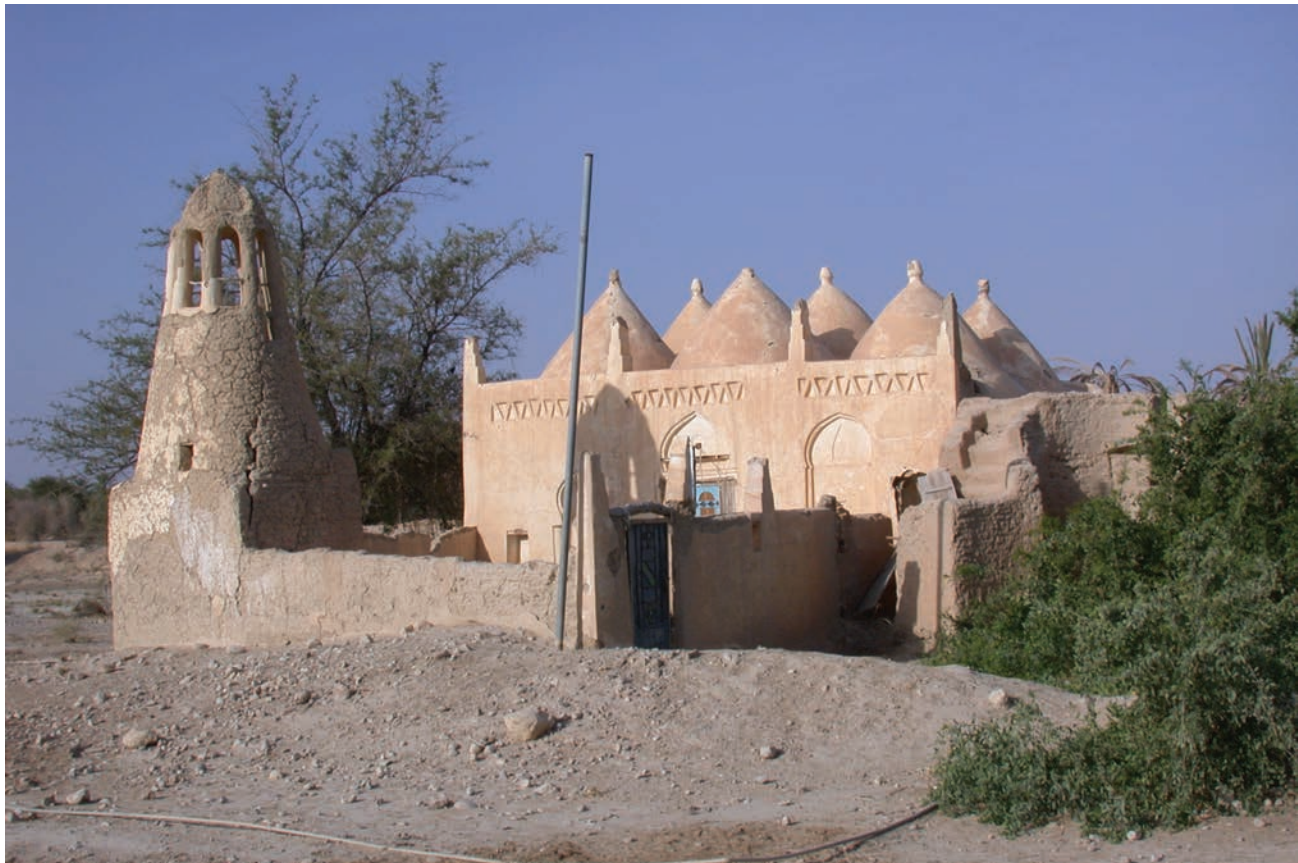
Figure 1.5. Mosque at Ghayl Bin Yumain. Photograph by Joy McCorriston.
