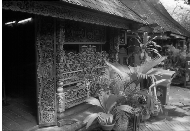
Figure 2-11 Example of porous wall construction in Java, Source: Author's collection.
