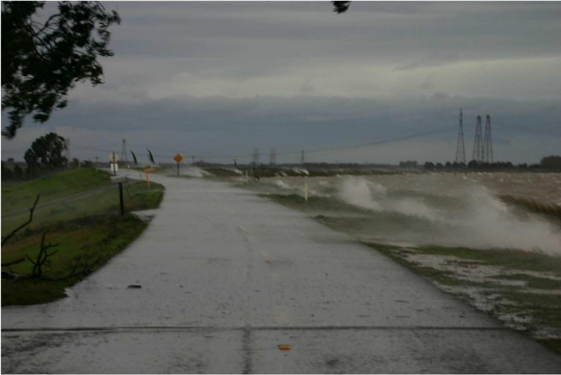
Figure P.1: Overtopping of levee, taken on Jan. 1, 2006 on Sherman Island levee adjacent to the San Joaquin River during high winds and High tide.
