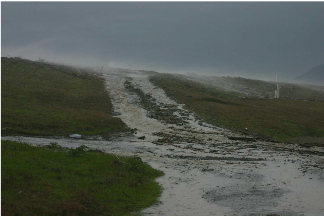
Figure P.4: Overtopping of levee, taken on Jan. 1, 2006 on Sherman Island levee adjacent to the San Joaquin River during high winds and High tide (land side)
