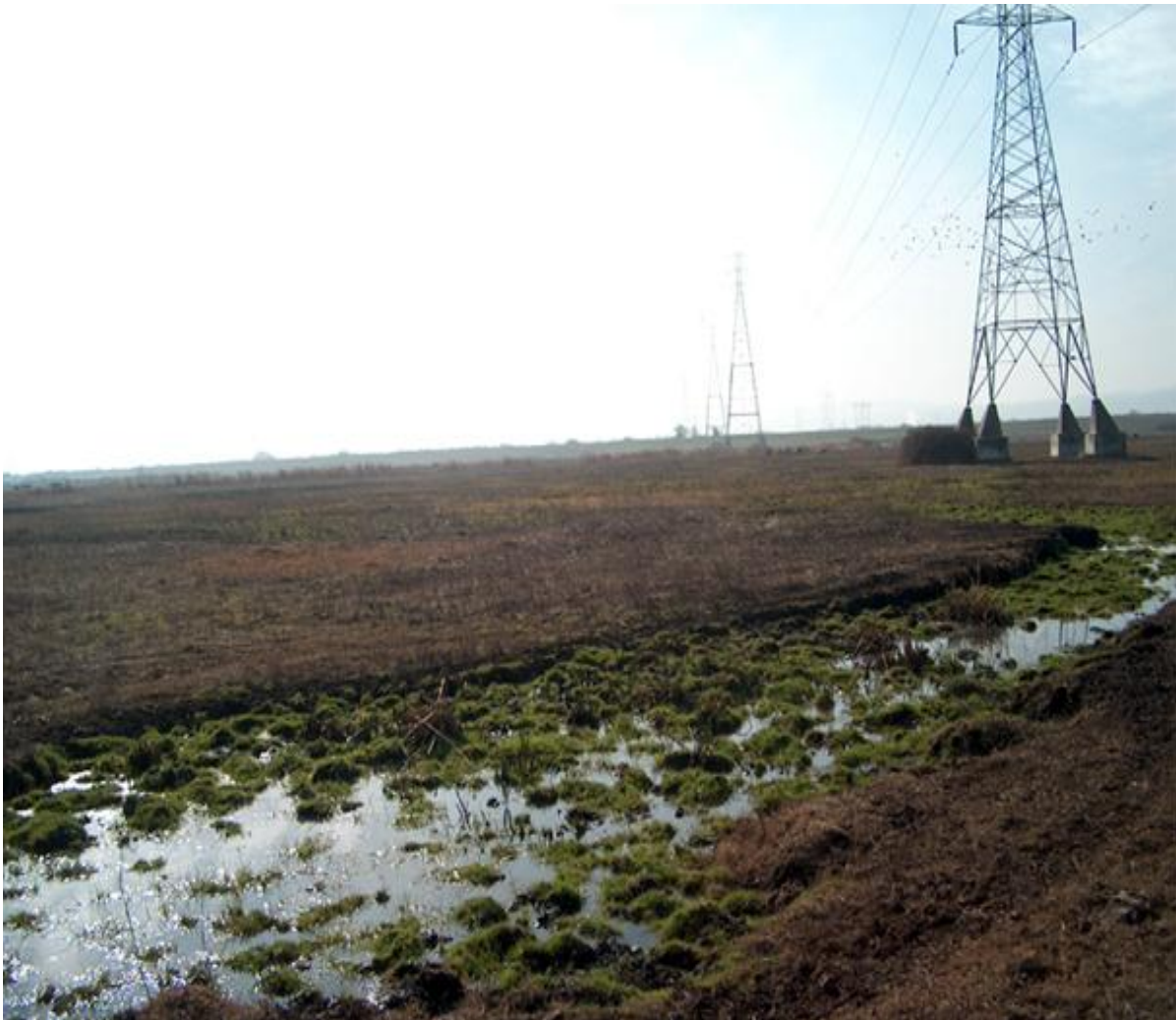
Figure 7-5: Transmission lines greater than 500kV cross Sherman Island. RESIN Sherman Island Pilot Project 2009
