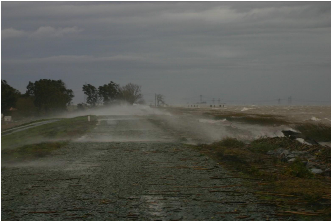
Figure P.2 Overtopping of levee, taken on Jan. 1, 2006 on Sherman Island levee adjacent to the San Joaquin River during high winds and High tide.
