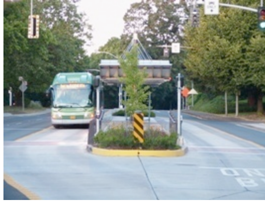
Figure 2-1 An Example of a Bus Stop in the BRT System with a Single Dedicated Lane
