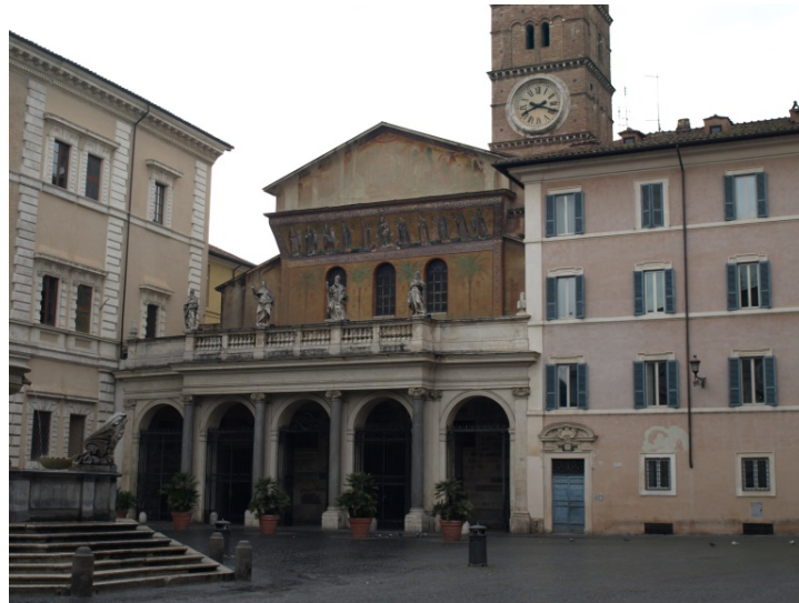
Fig. 5. Santa Maria in Trastevere, façade. Photo: author.
