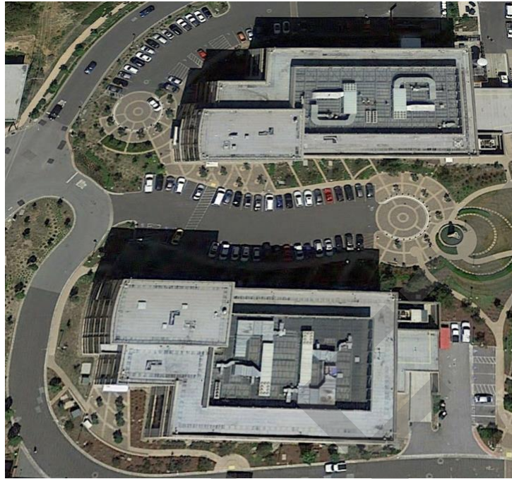
Top view of Building A (top) and Building B (bottom).
