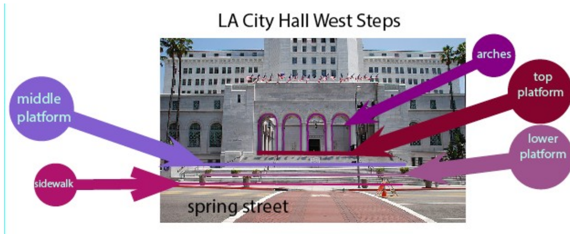
Figure 30. West steps platforms and arches.
