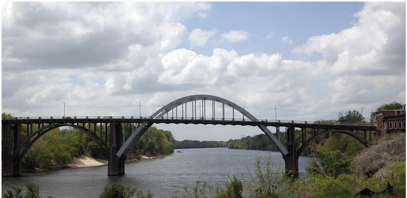
Edmund Pettus Bridge, Selma, Alabama, 2010. CAROL M. HIGHSMITH/THE GEORGE F. LANDEGGER COLLECTION OF ALABAMA PHOTOGRAPHS IN THE CAROL M. HIGHSMITH ARCHIVE, LIBRARY OF CONGRESS, PRINTS AND PHOTOGRAPHS DIVISION
