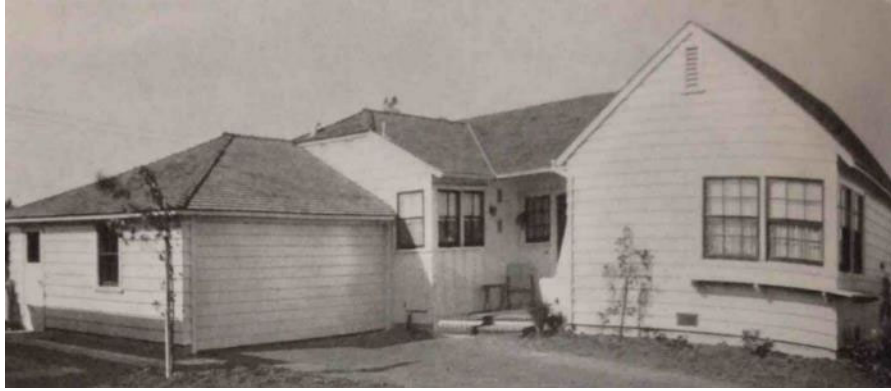
Figure 4.19. Front elevation of two-bedroom ranch modeled on Dailey's LIFE House plan. Source: American Builder , October, 1941
