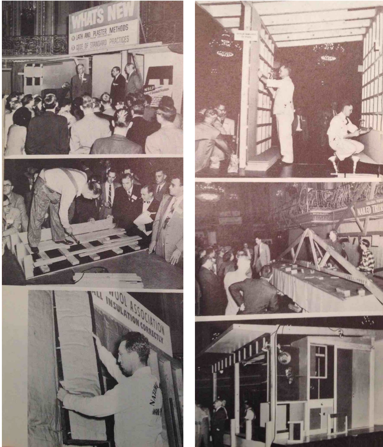
Figure 6.7. Scenes from six simultaneous demonstrations at the “How to Do It Circus” at the 1955 NAHB Convention at the Hilton Hotel, Chicago. Demonstrations included (left, top to bottom) lathe and plaster, applying strip hardwood flooring over concrete, installing mineral wool batting insulation, (right, top to bottom) applying insulated board roof decking, nailed truss construction, and hardboard siding installation. Source: NAHB Correlator February 1955, pages 24-25.
