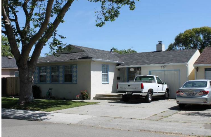
Figure 4.30. 16010 Paseo del Campo, San Lorenzo Village. Photograph Elaine Stiles 2016.
