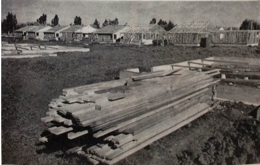
Figure 4.36. House load in place during construction at San Lorenzo Village. Source: LIFE , April 15, 1946.
