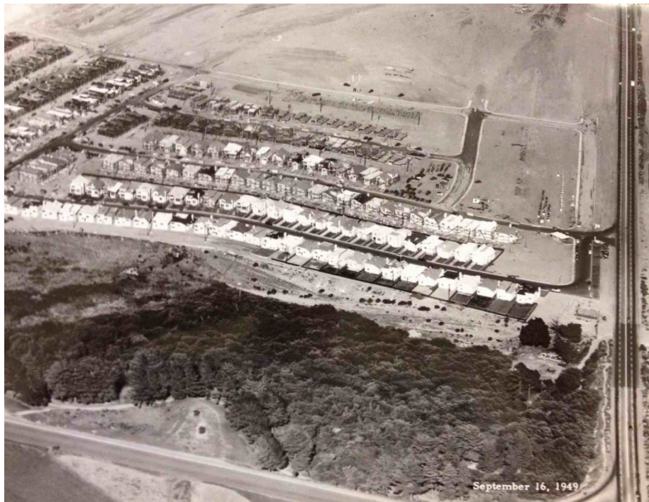
Figure 328. Aerial view of street layouts and lot sizes in the early phases of Westlake, 1949. Source: Daly City History Guild, Daly City, California.
