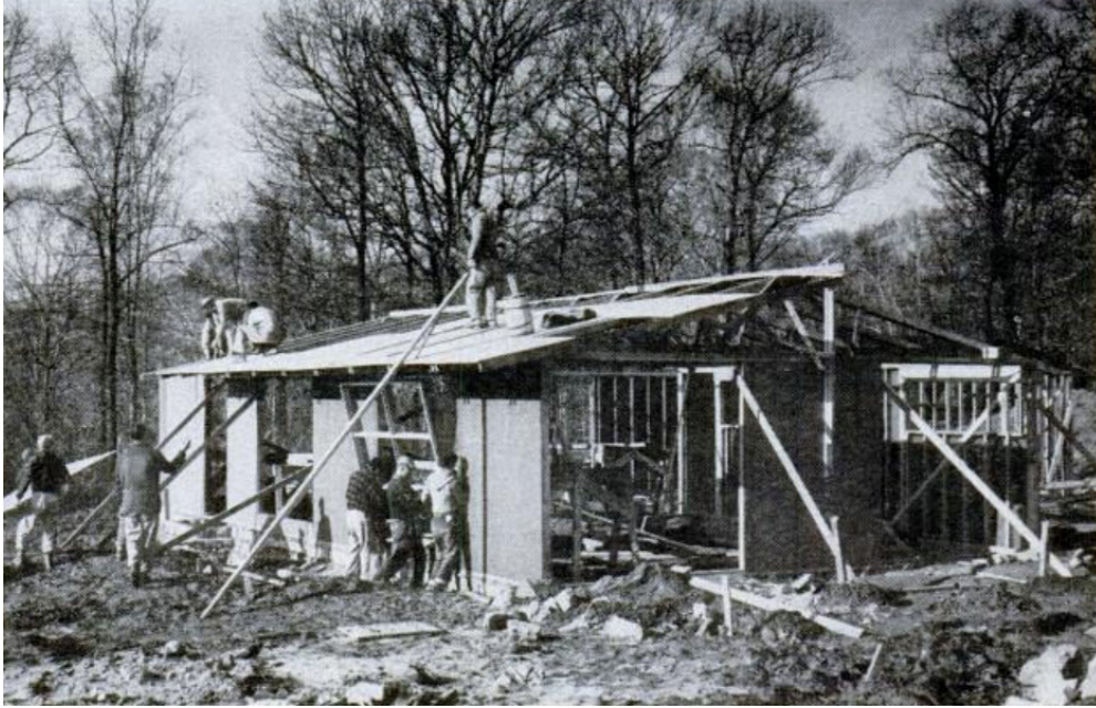
Figure 6.19. Workmen setting in preassembled window units and attaching pre-cut roof sheathing in a Wallace Arters' Lima, Pennsylvania Trade Secrets House model. Source: LIFE, January 5, 1953, page 14.
