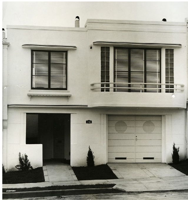
Figure 3.17. Example of Doelger's "Styleocrat" model, constructed in 1941 in the Sunset. Source: Western Neighborhoods Project.
