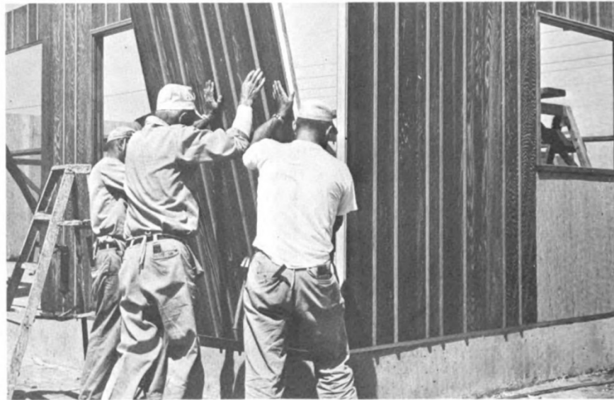
Figure 15—Placing exterior wall panel
