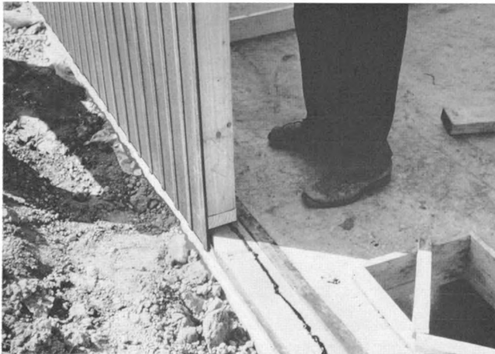
Figure 9—Masonite panels extend about 2½" below base plate
