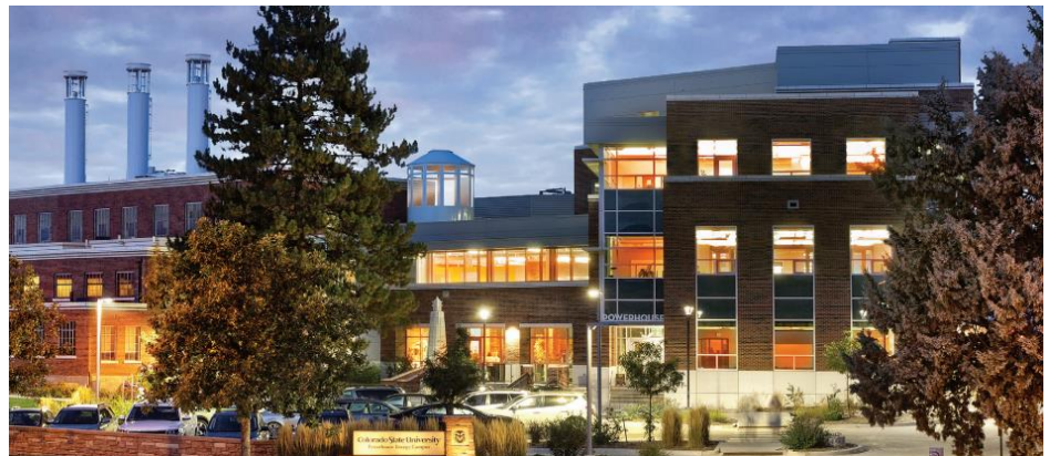
Photo: Fort Collins Utilities' Integrated Design Assistance Program.
