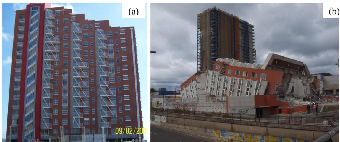
Figure 4-1. Torre Alto Rio (a) before, (b) after the earthquake [(a) Bonelli, 2010; (b) Wallace, 2010]
