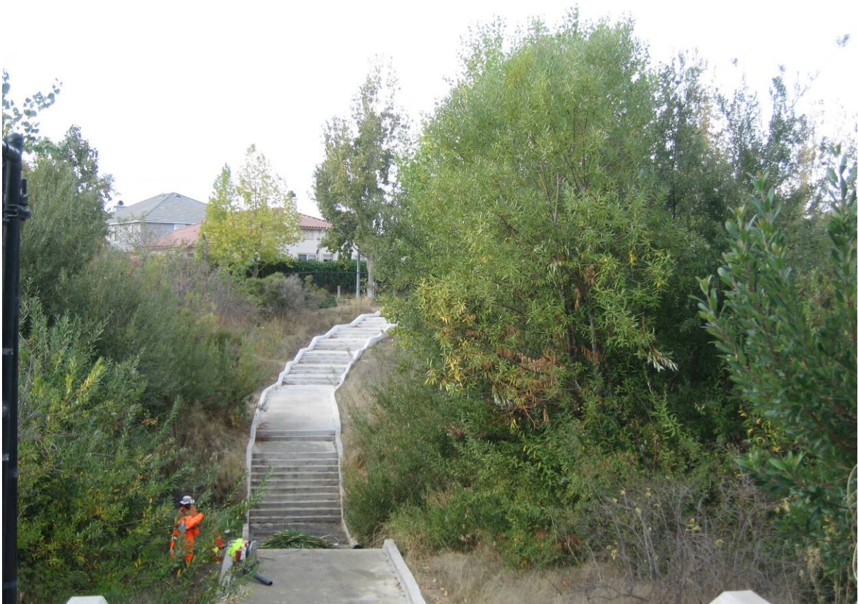
Figure 10: Annual Maintenance at the Pedestrian Walkway (Reach 2, Right of Bank)
