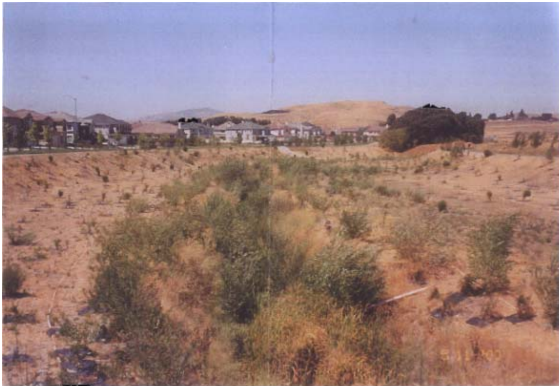
Upstream View to North of Central Parkway Bridge
