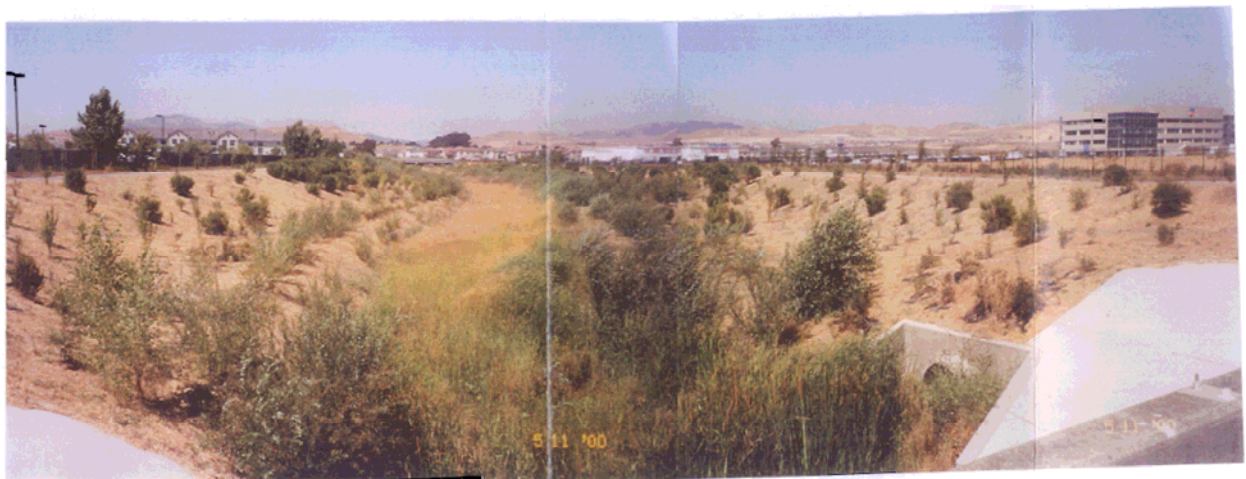
Upstream View to North From Highway 580 Bridge
