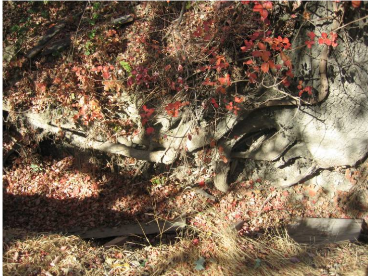
Figure 6: Oak Tree Roots Exposure
