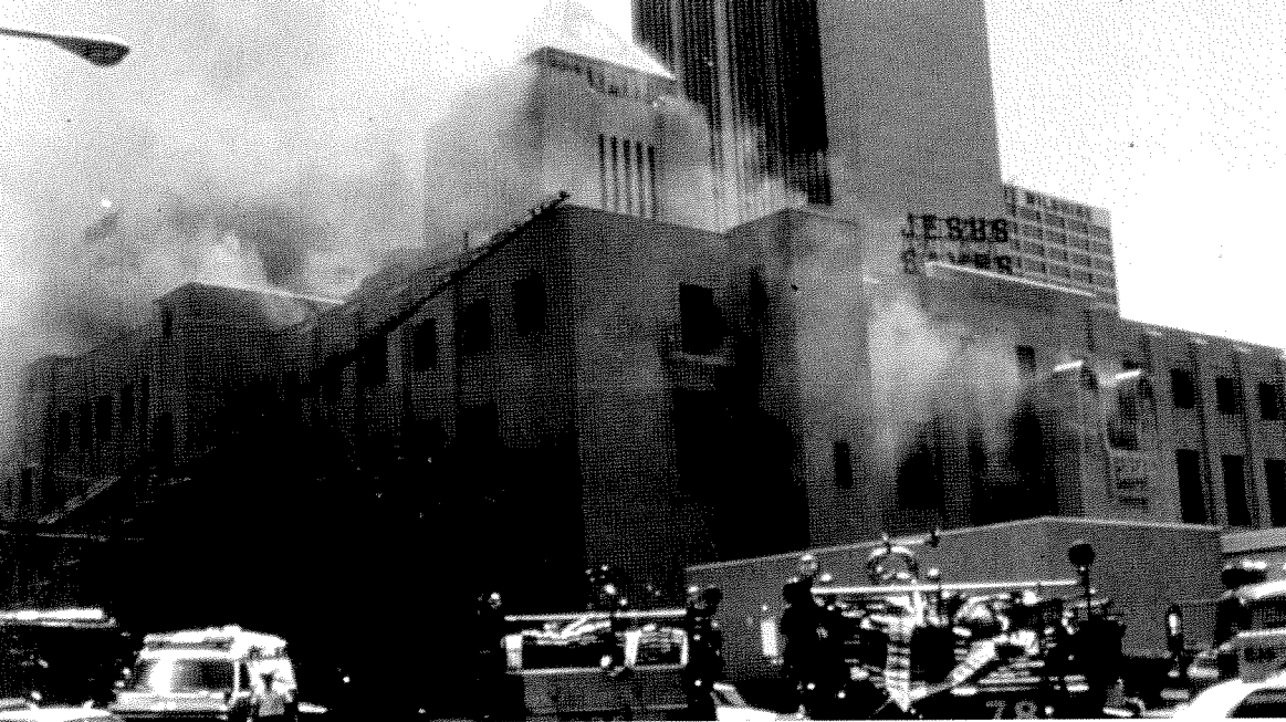
top: Library on fire as a result of arson, 1986.
