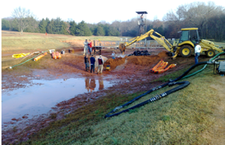
Figure 5.28: Test levee under construction.
