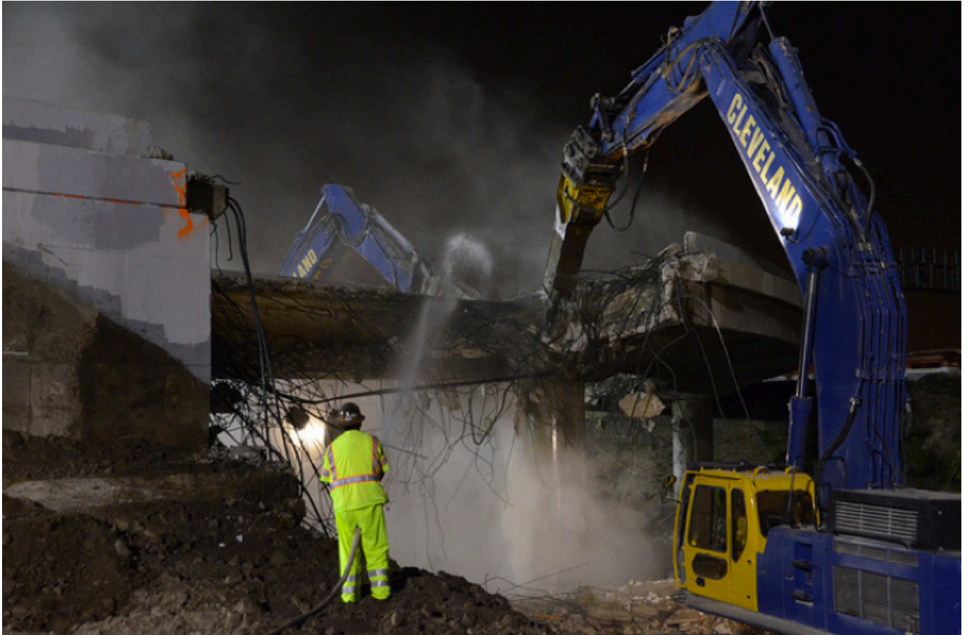
Figure 4.8: The final left-exiting off-ramp is destroyed in February 2012. 109
