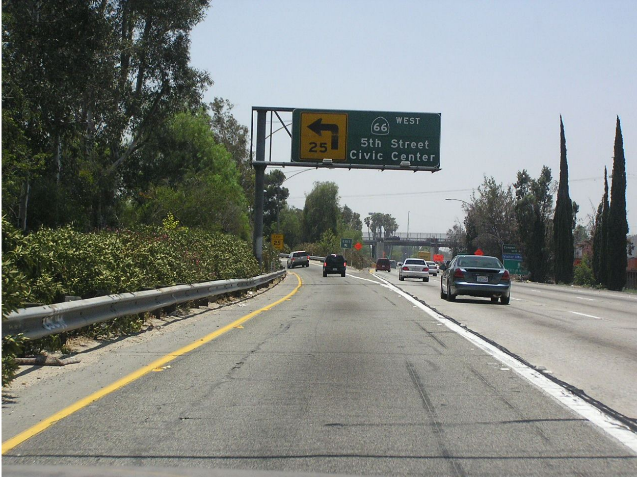
Figure 4.7: The 5 th Street left-exiting off-ramp is shown here on the southbound lane of the I-215 freeway in 2002. This off-ramp led motorists into the eastern end of the city with no convenient access into the west end of San Bernardino. Route 66 would later be re-routed into downtown off of Mt. Vernon Avenue, obscuring the west side's ties to the iconic highway. 108
