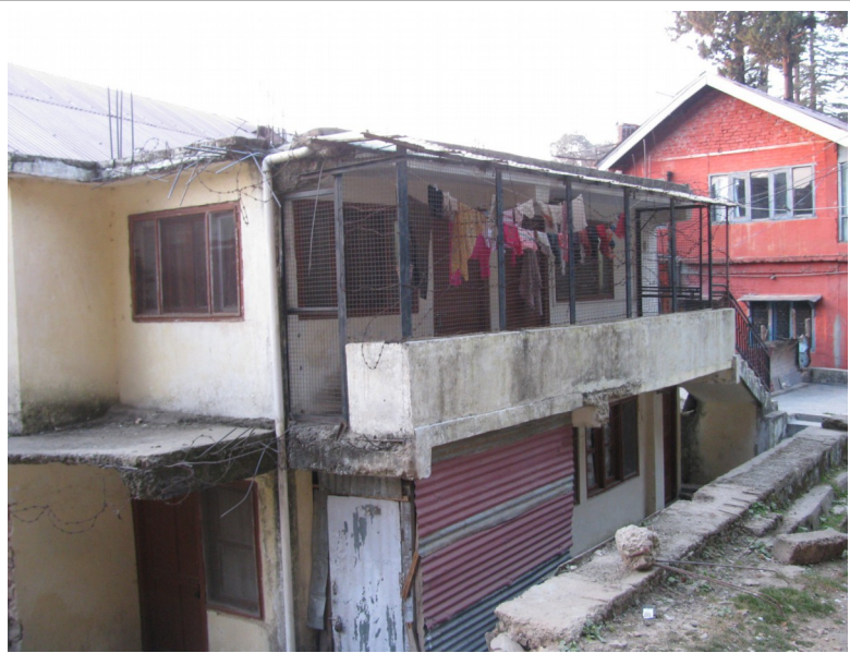
Figure 44. Caged house on Jakhoo Hill. One of many monkey-proofed homes around Shimla. There are many houses in the monkey-bearing neighborhoods of Varanasi, Vrindavan, Delhi, and Bundi with similar caged porches.
