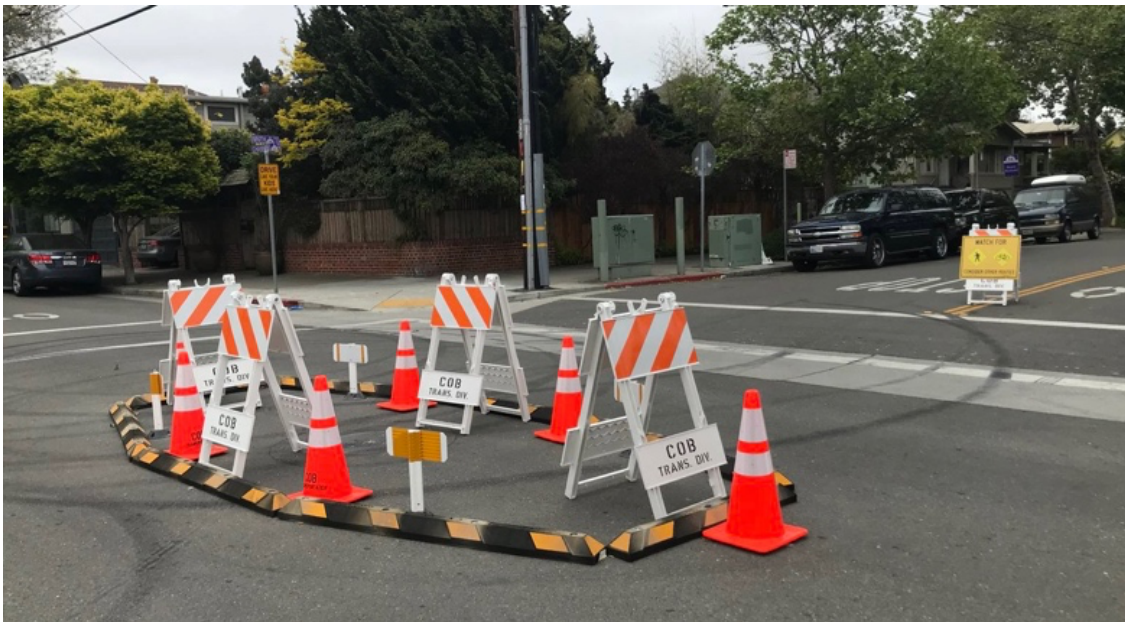
Figure 12: Traffic diverter to support slow vehicle speeds along designated Slow Streets in Berkeley. Source: Berkeley Transportation Division
