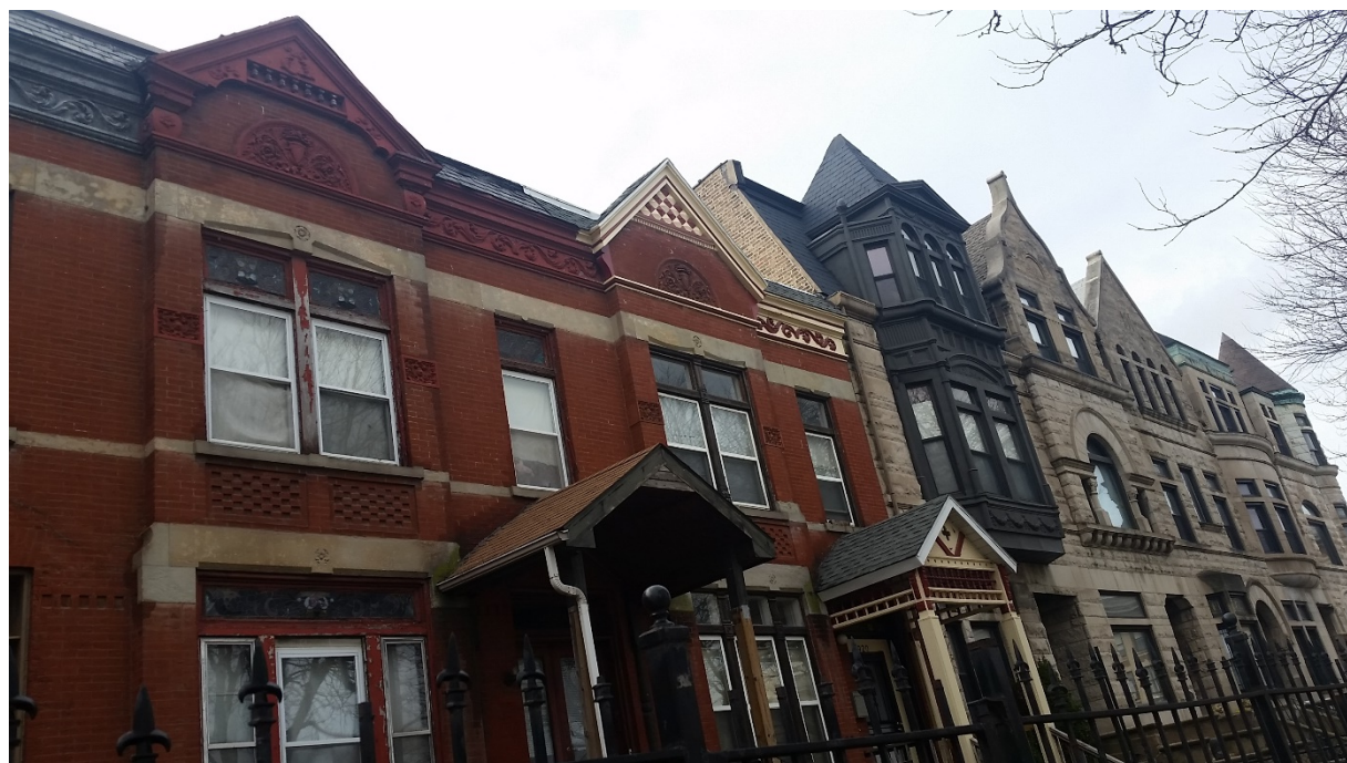
FIGURE 5.2 Homes across from vacant lot, South Prairie Ave near E. Pershing Rd, Chicago, IL, taken by author, March 2017
