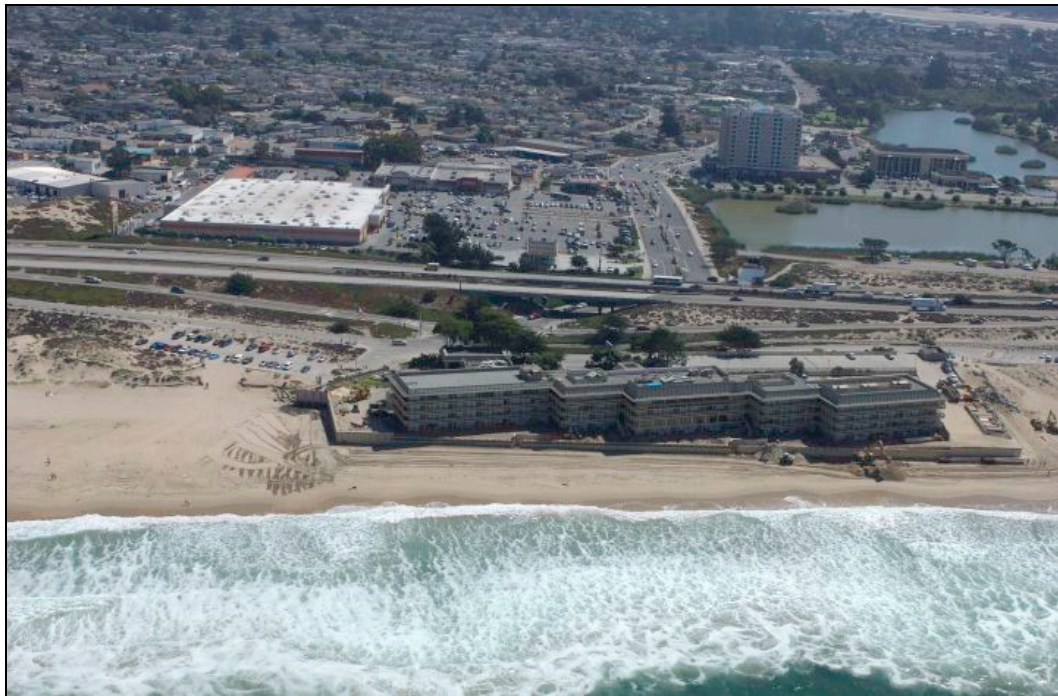
Fig. 1.2: The Best Western Hotel Beach Resort and seawall in Monterey showing passive erosion and severe placement loss of the beach (photo by Kenneth and Gabrielle Adelman)
