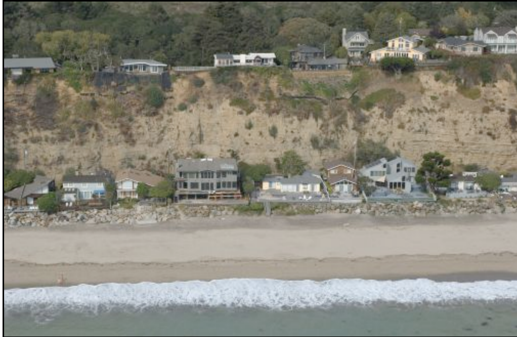
Fig. 1.27: Class V shoreline at New Bright State Beach in Central California. The high classification is due to the presence of infrastructure not only on the bluffs, but also on the back beach fronted by coastal armoring (rip-rap) (photo by Kenneth and Gabrielle Adelman)
