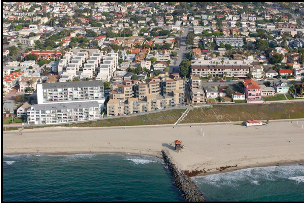
Fig. 2.17: Aerial photo of the Redondo Beach Topaz Street groin and back-beach development (photo by Kenneth and Gabrielle Adelman)
