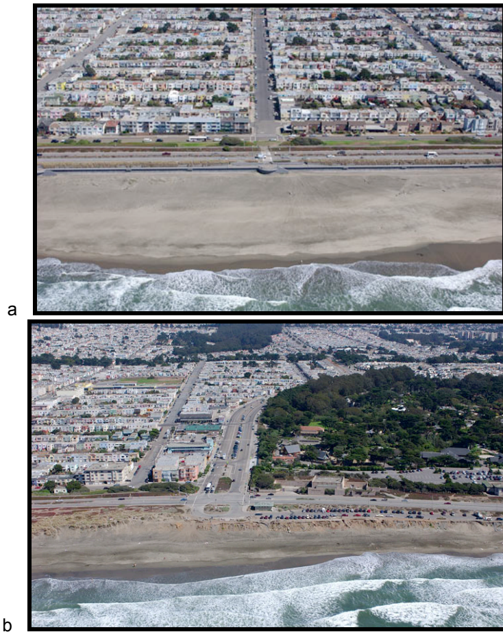
Fig. 2.50: (a) Aerial photo of Ocean Beach bounded in the backshore by the Ocean beach seawall and the Great Highway (b) Ocean Beach at Sloat Blvd, characterized by high rates of erosion (photos by Kenneth and Gabrielle Adelman)
