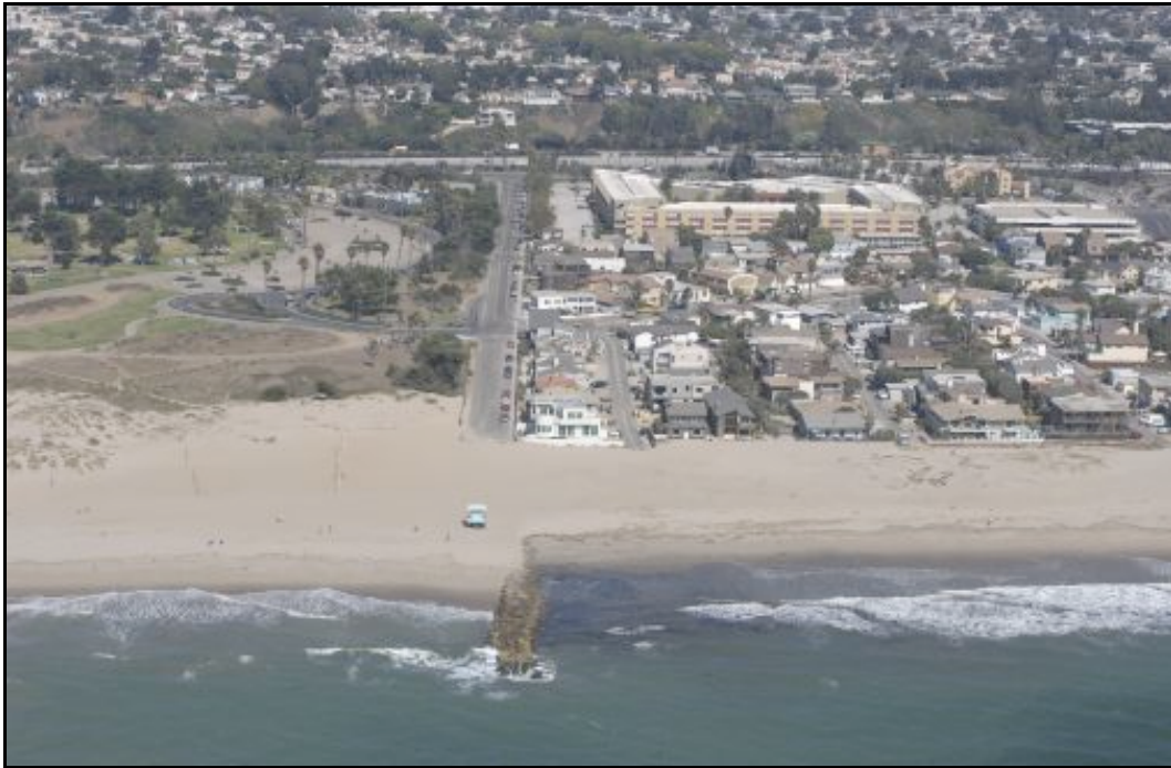
Fig. 1.29: San Buenaventura State Beach (left of the groin) directly adjacent to Ventura public beach (right). Although the presence of the groin has widened the state beach, it is clear in comparing the back beach extents that back-beach development on the public beach side has contributed to beach narrowing and placement loss (photo by Kenneth and Gabrielle Adelman)
