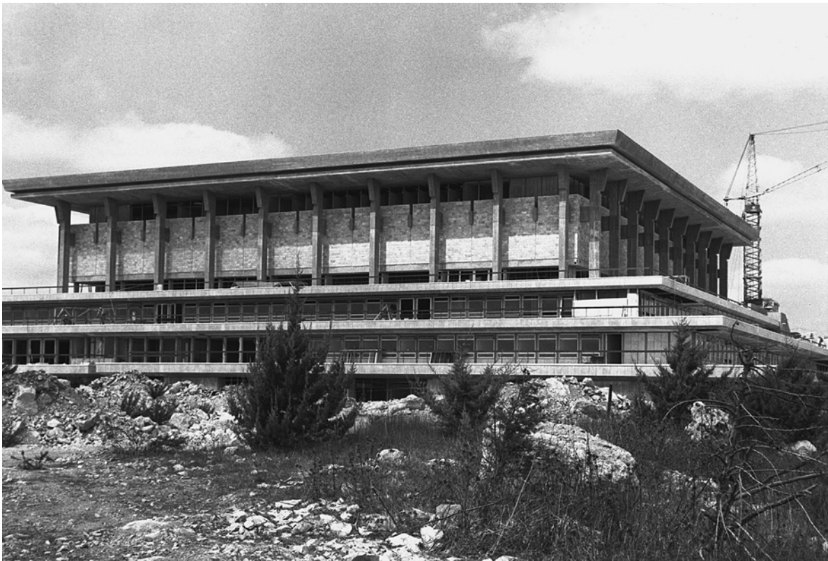
FIGURE 1.4 The Knesset under construction, Jerusalem, early 1960s. Photograph: Moshe Fridan, Israel Government Press Archive.
