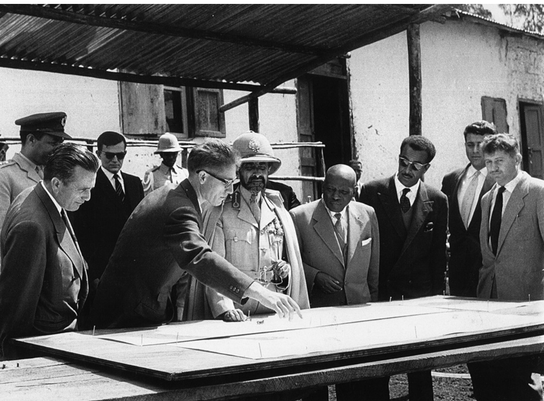
FIGURE 5.2 Zalman Enav explaining a building plan, 1960. Foreground, from left to right: Hannan Bar-On (Israel’s consul general in Ethiopia), Zalman Enav, Haile Selassie, Menasse Lemma (director general of the Ministry of Finance), Michael Tedros, Solel Boneh engineer Yehoshua Greunspan, and Solel Boneh project manager Dov Eisenberg. Courtesy of Zalman Enav.
