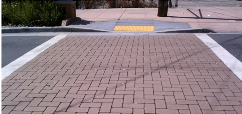
Figure 10. Concrete crosswalk imprinted to resemble permeable pavement
