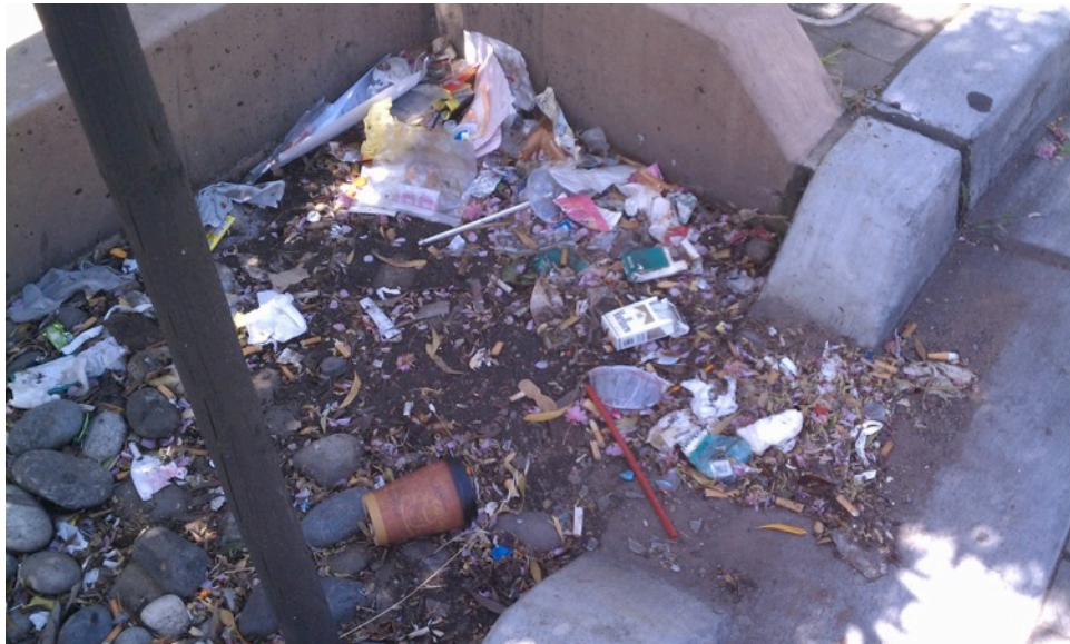
Figure 14. Trash collecting at a planter stormwater inlet
