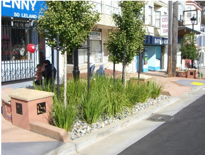
Figure 7. Bioretention planter with no stormwater inlet
