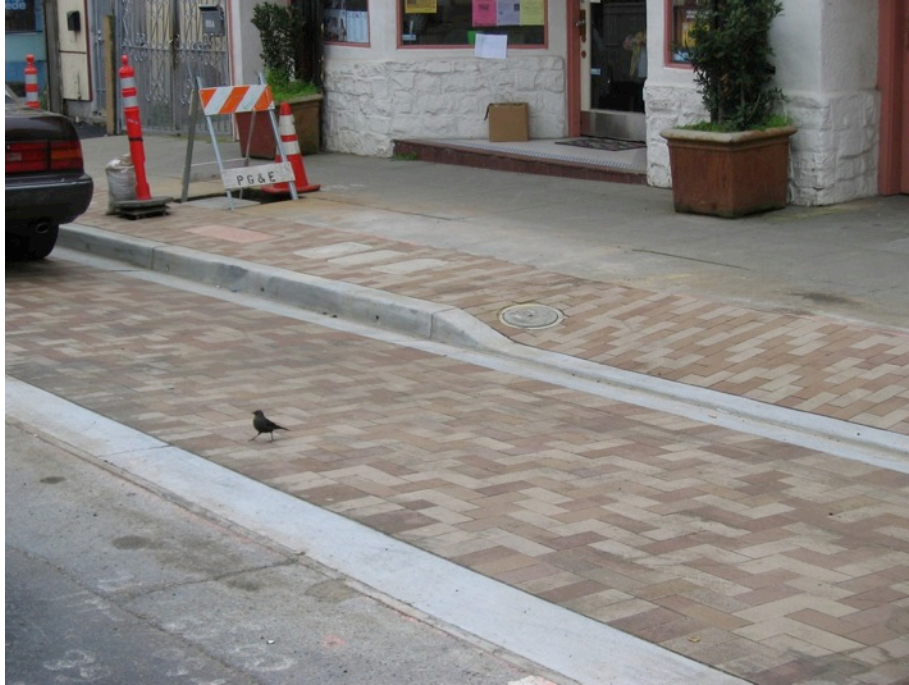
Figure 4. Permeable pavement on sidewalk and parking strip
