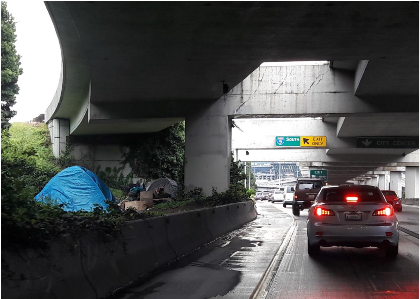
Figure 1. Tents Next to a Highway
