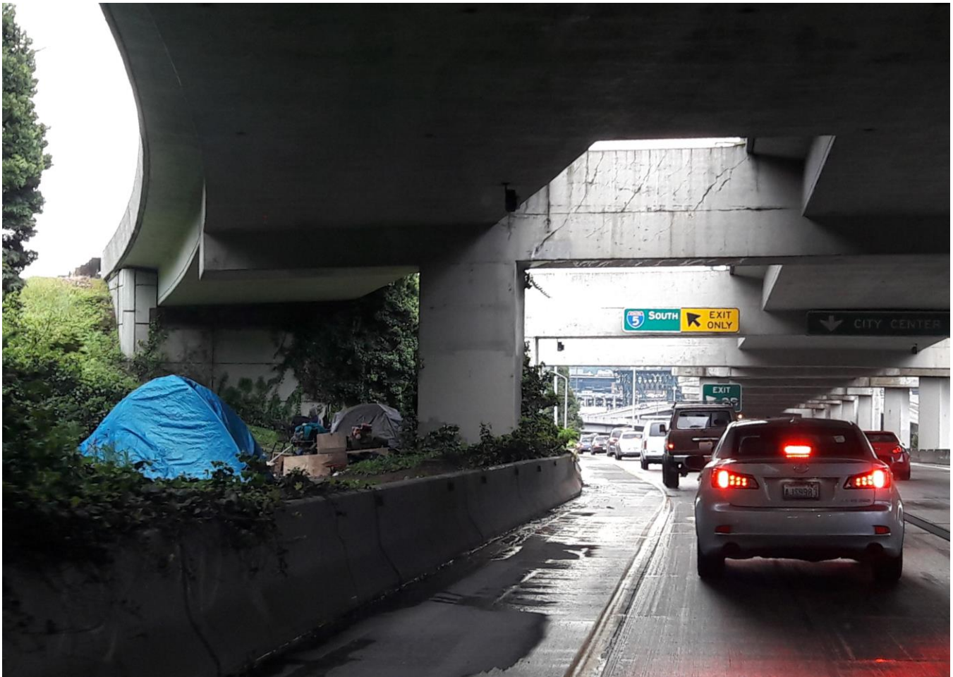
Figure 1. Tents Next to a Highway
