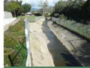
The urban watershed of the estuary includes trapezoidal concrete channels which create flashier rain events and offer few opportunities for water to soak into the water table.
