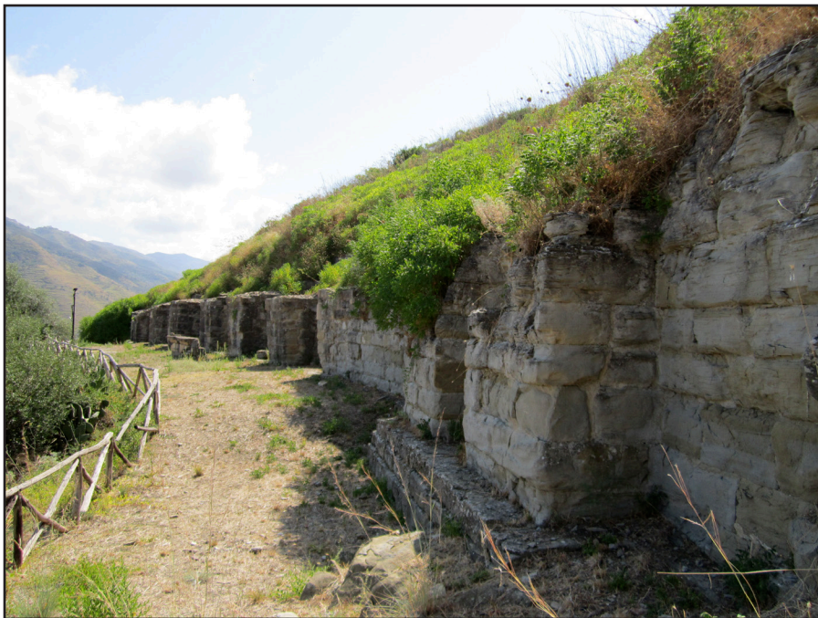
b. Halaesa: the “counterforts” on the northeastern slope of the Santa Maria delle Palate hill.
