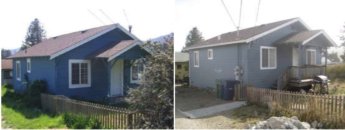
Image 14 - P5 Pre- and Post-Retrofit
