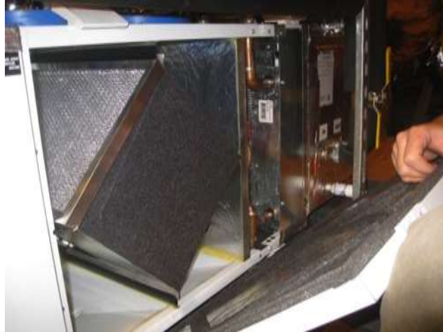
Image 5 - P2 Passive HRV Core Integrated with Attic Air Handler
