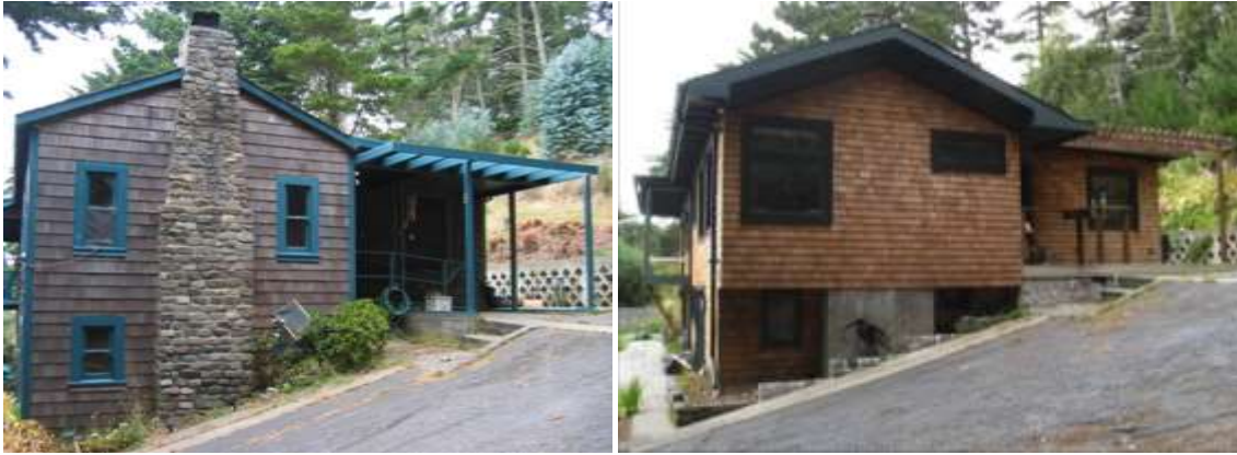
Image 43 - P10 Pre- and Post-Retrofit
