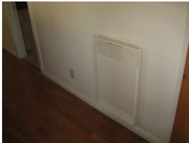
Image 17 - P5 Electric Resistance Wall Heater
