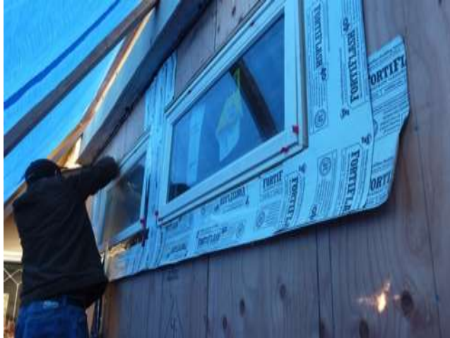
Image 32 - P7 Installation of New Window Flashing on Rear-L
