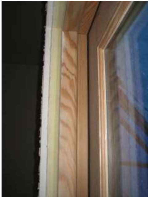
Image 31 - P7 Rear-L New Windows, Interior Continuous Foam Board and Sheetrock
