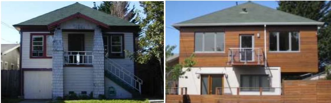
Image 1 P1 Pre- and Post-Retrofit
