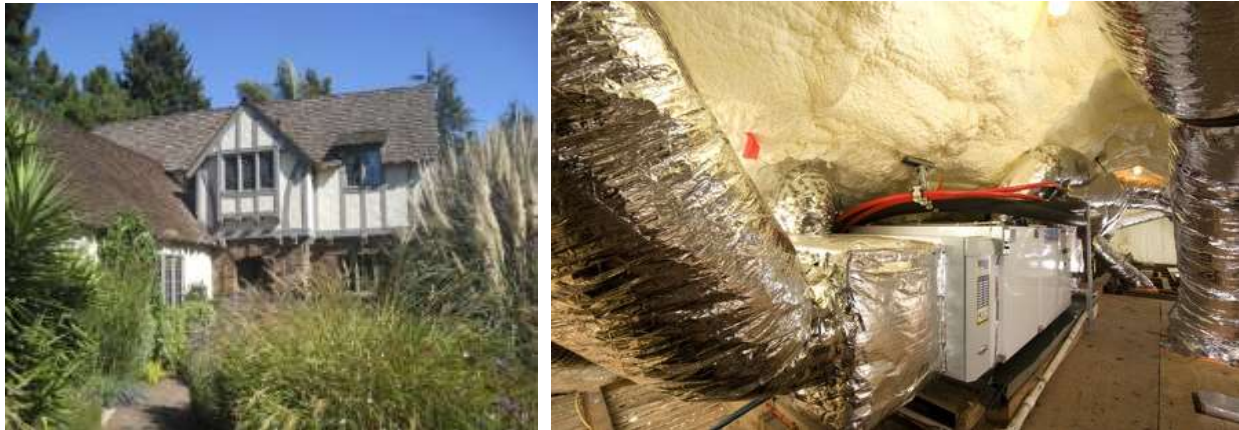
Image 3 - P2 Post-Retrofit Exterior and Insulated Attic
