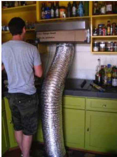
Image 24 - P6 North, Kitchen Range Hood Airflow Measurement
