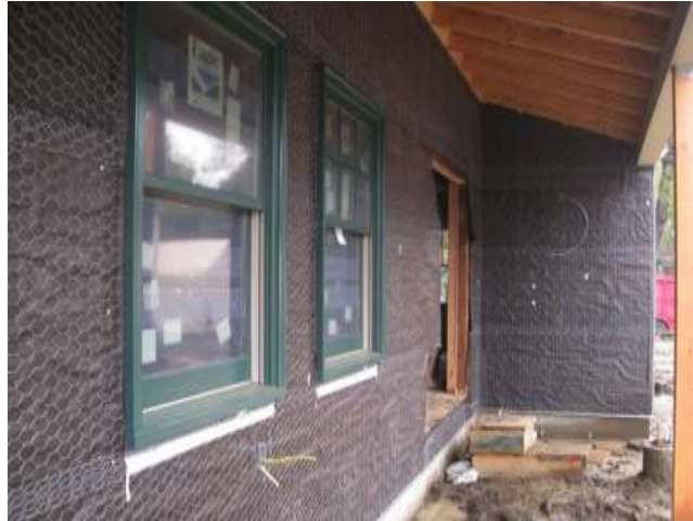
Image 21- P6 North, New Tar Paper WRB and Windows, with Plaster Lathe
