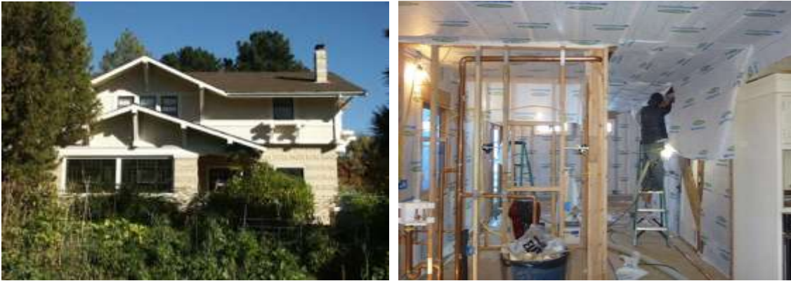
Image 28 - P7 Front of Home and House-Within-A-House Insulating
