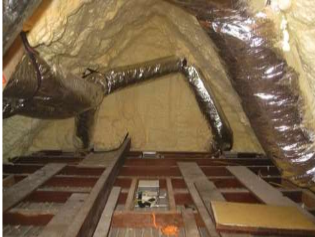
Image 4 - P2 Spray Polyurethane Foam in Sealed Attic
