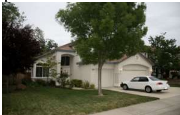
Image 39 - P9 Post-Retrofit Exterior
