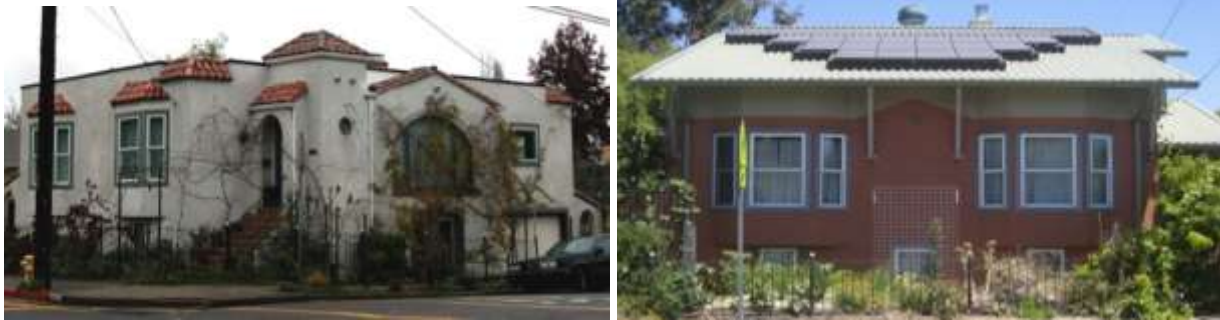
Image 10 - P4 Pre- and Post-Retrofit
