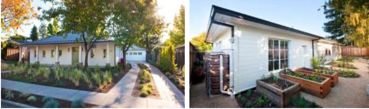
Image 9 - P3 Post-Retrofit Front (left) and Rear of Home (right)
