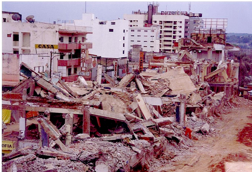
Figure 33. Demolition of a Futuro gallery for the Pilot Plan upgrades
