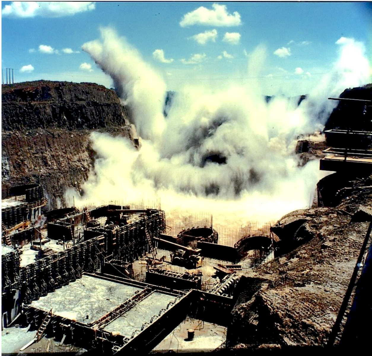
Figure 11. An explosion for the construction of the Itaipú Hydroelectric Dam
