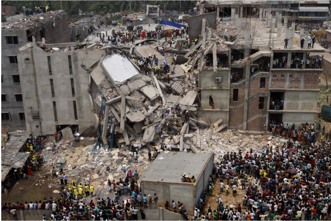
Figure 1.2: Rana Plaza building collapse
