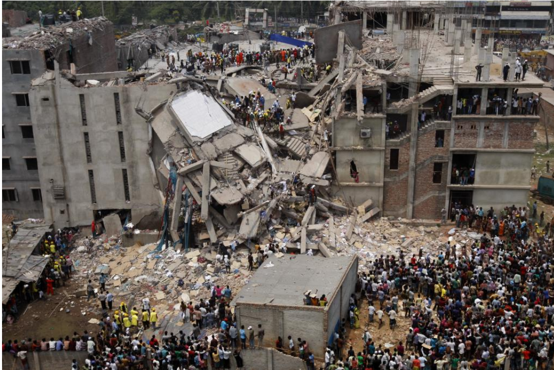
Figure G1: Rana Plaza factory complex collapse
