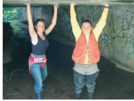
Lorraine and Sarah hold up the culvert leading to 8-ft cement steps
