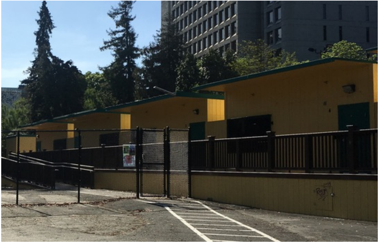
Image 4: The New Temporary Mosswood Recreation Center
