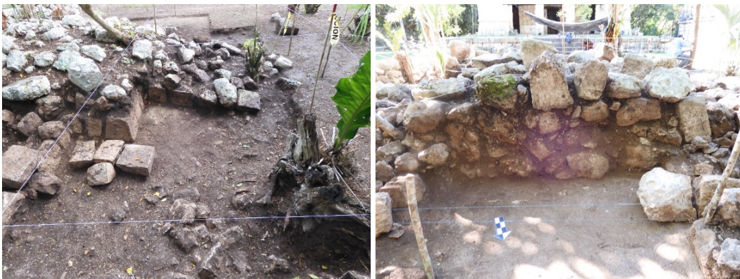
Figure Appendix D.3 a) Corners in situ. b) North view of the masonry box inside the Str. 5C13 after the removal of the north stairways.
