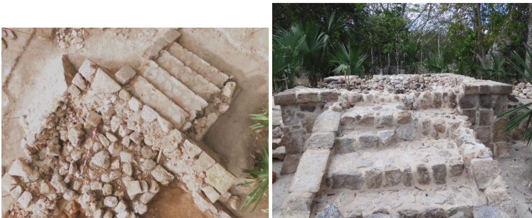
Figure Appendix D.4 a) Plant view of the consolidation process of the north and west stairs. b) East staircase showing the use of plaster and fill when there were no carved rocks.
