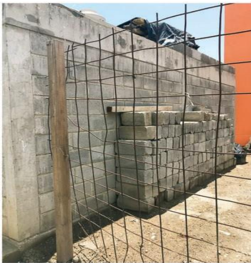
Figure 3. Bricks pulled from the rubble of a fallen structure, cleaned for reuse.
