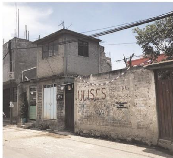
Figure 4. A home in San Gregorio with an autoconstructed second story.
