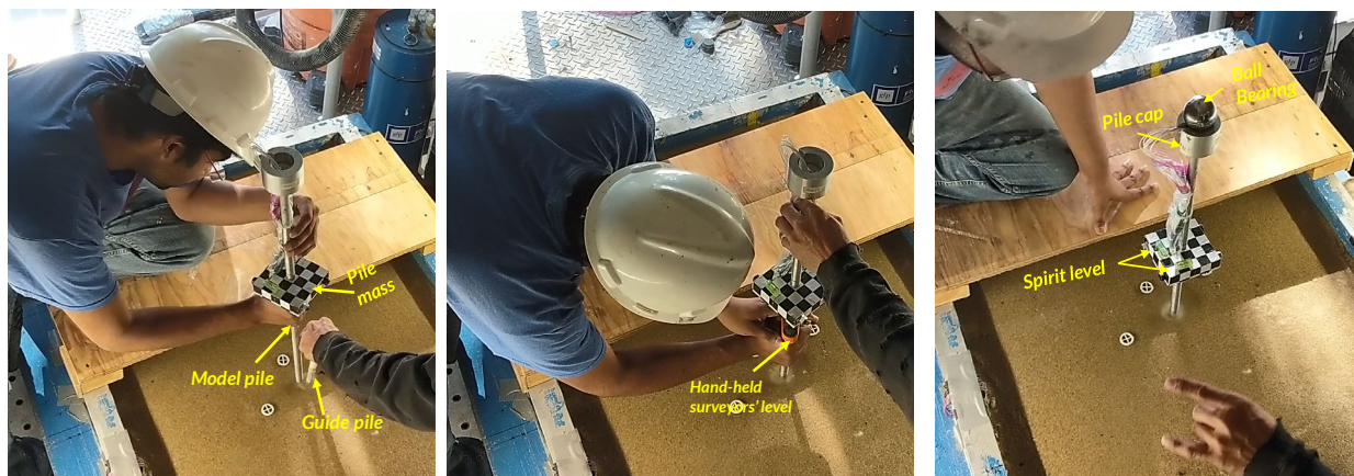
Removing the guide pile
