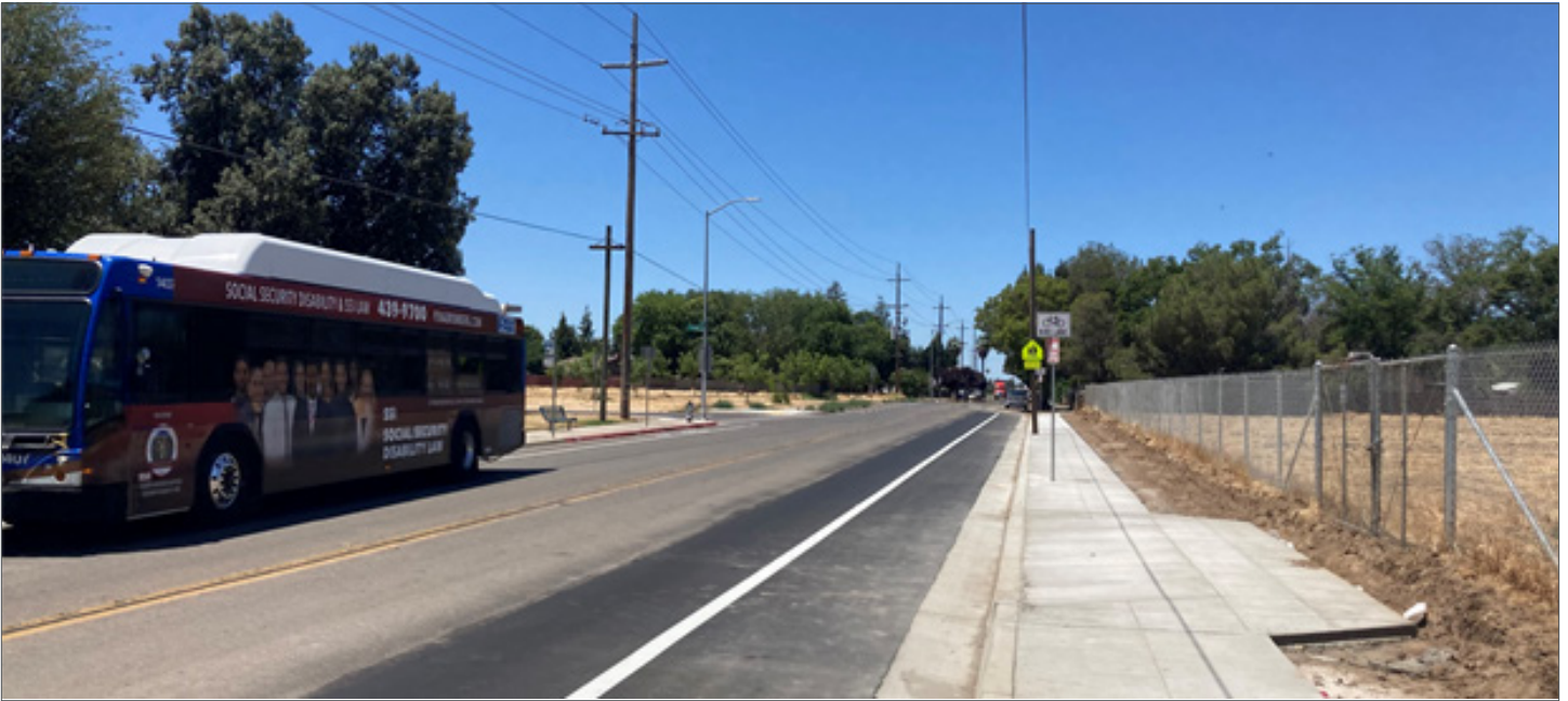
A Class II bicycle lane long Annadale Avenue. Photo credit: Self-Help Enterprises
