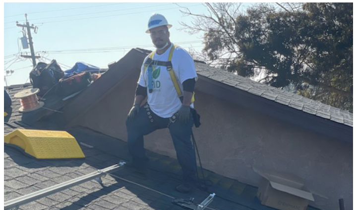
Matthew De La Rosa working at installation project job sites in Fresno. Photo credit: GRID Alternatives
