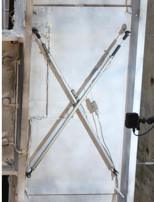
Figure 4.89 Specimen C7: Doubler Plate at End of Test
