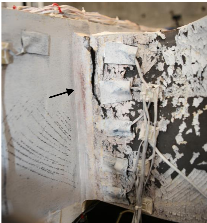
Figure 4.127 Specimen W2: East Beam Top Flange Partial Fracture during Excursion to -0.06 rad (2 nd Cycle)
