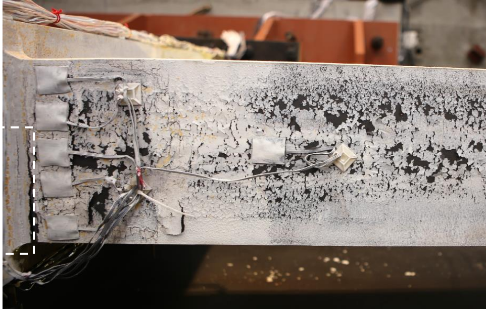
Figure 4.170 Specimen W4: East Beam Top Flange CJP Weld Fracture at -0.04 rad (2 nd Cycle)
