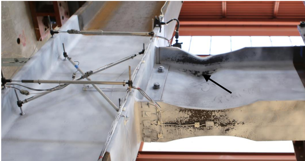
Figure 4.21 Specimen C4: Beam Web Buckling at -0.04 rad (1 st Cycle)
