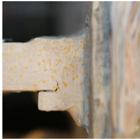
(b) Weld Fracture
