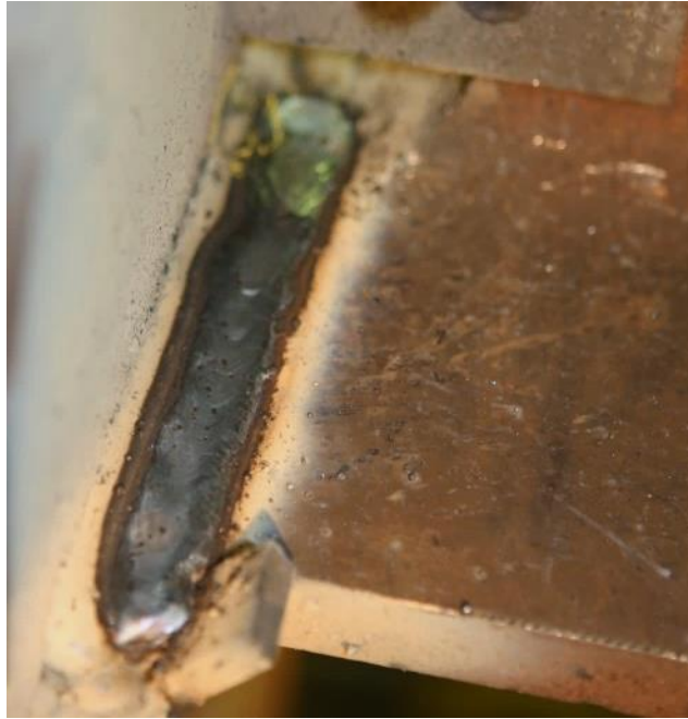
(a) Beam Bottom Flange
