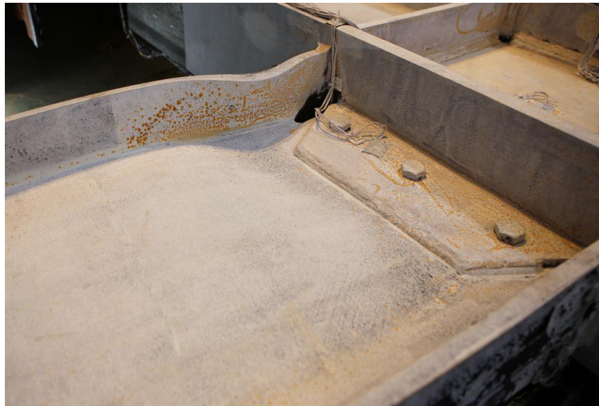
Figure 4.169 Specimen W4: West Beam Web Buckling at +0.04 rad (1 st Cycle)
