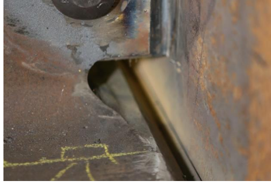
(b) Weld Access Hole
