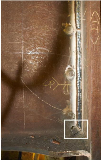
(a) Completed Weld
