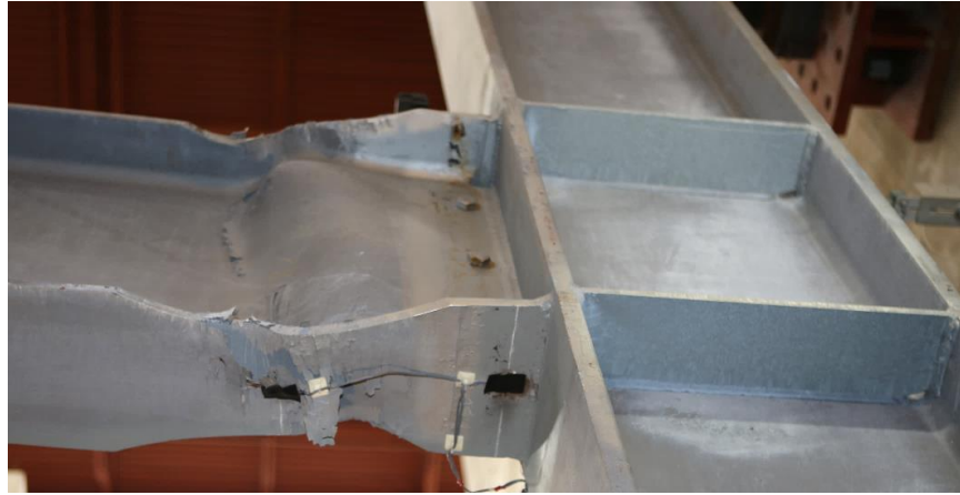
Figure 4.67 Specimen C6-G: Web Local Buckling
