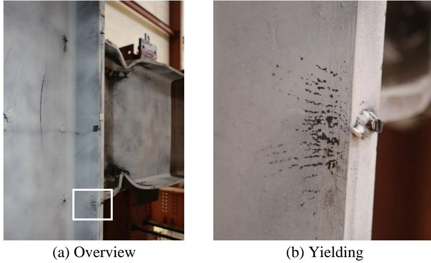
Figure 5.13 Specimen C4: Observed Column Flange Localized Yielding (End of Test)
