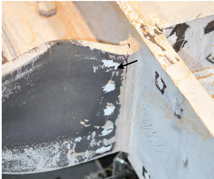
Figure 4.153 Specimen W3: West Beam Top Flange (End of Test)
