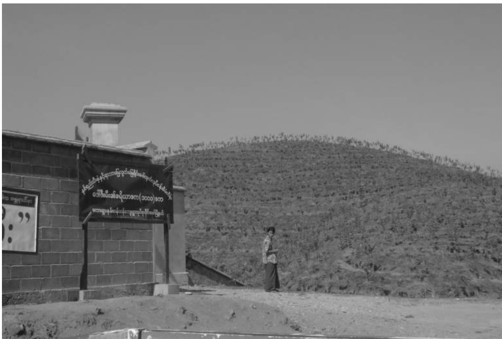
Figure 10. A brick wall in “Chinese style” greets outsiders to a private rubber concession, details posted on the official government sign, near Nam San Yang, Kachin State. Source: author.
