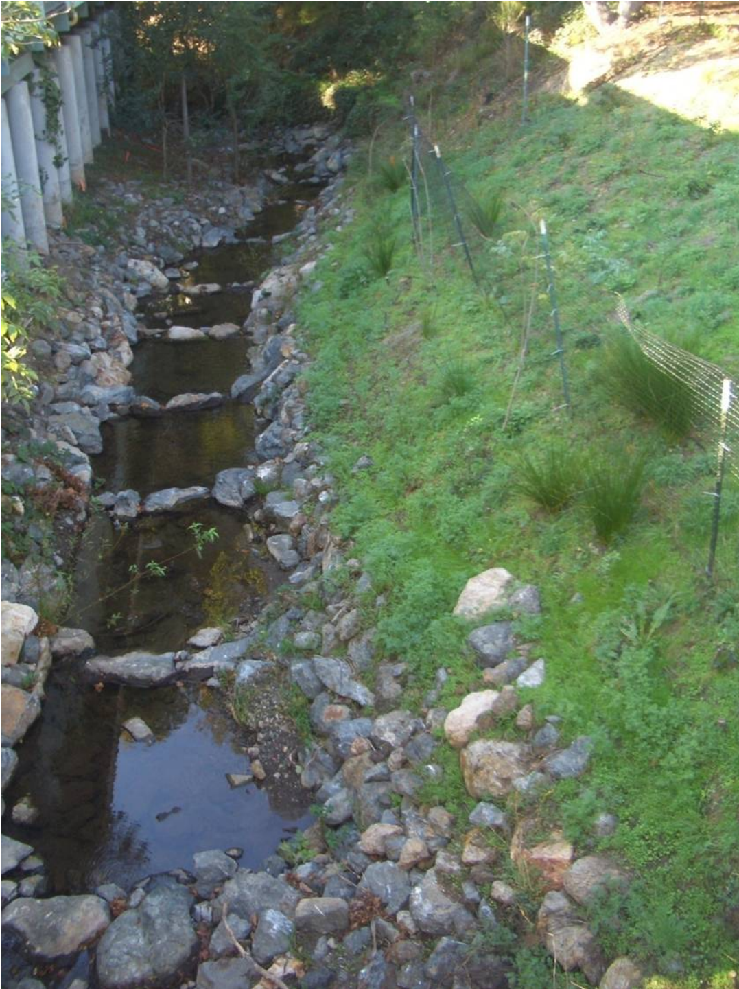
Figure 11. Step Pools installed as part of CCWRAP Phase II
