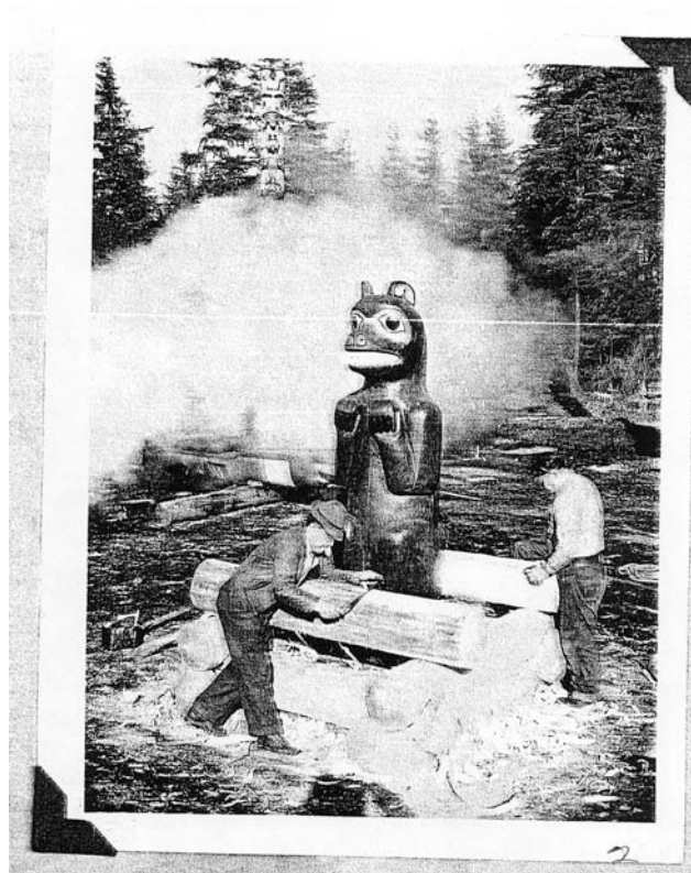
Fig. 1.23 Building cribs for base of poles, Hydaburg totem park (USFS Historical Photograph)
