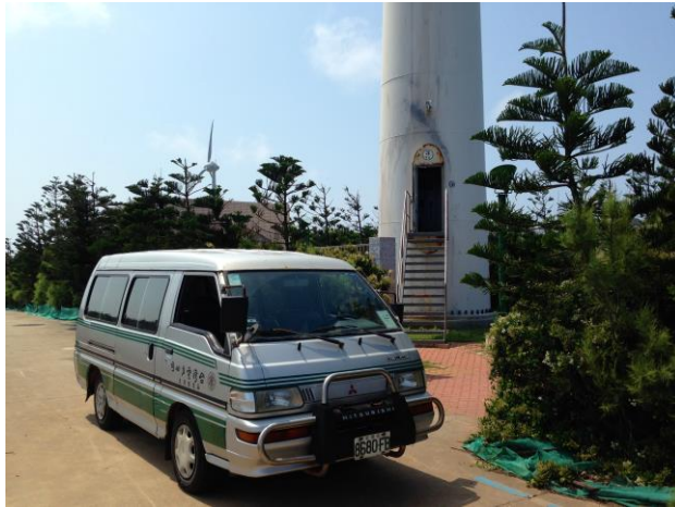
Figure 4-3. Taipower's Vehicle Dispatched for the Maintenance of Wind Turbines. Photo by author.
