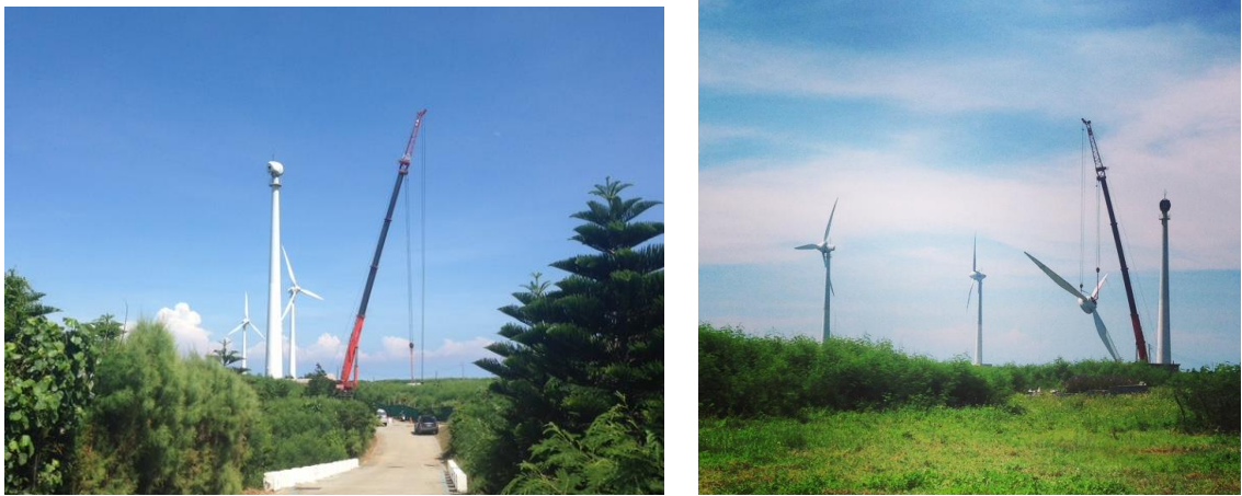
Figure 4-4. Repair Work for Broken Wind Turbines. Photo by author.
