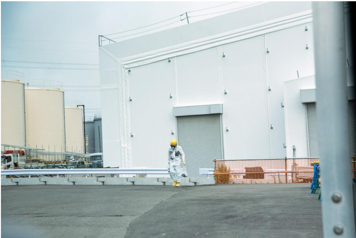
Figure 82: A lone worker inside the power plant (7/11/2016)
