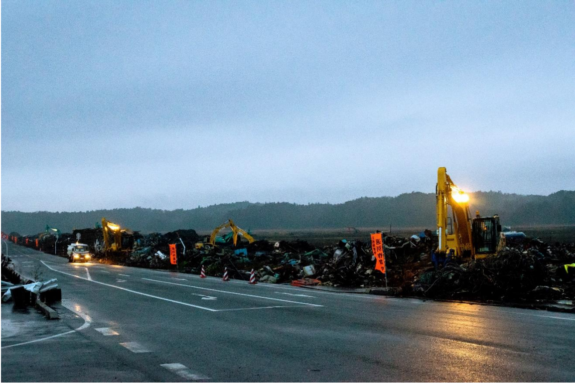
Figure 52: Debris cleanup for coastal zone in Namie begins in 2014 (12/17/2014)
