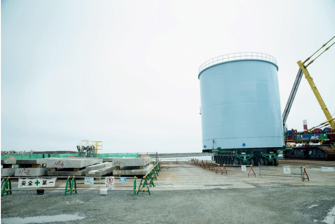
Figure 81: Huge liquid container tanks are transported inside the power plant (7/11/2016)
