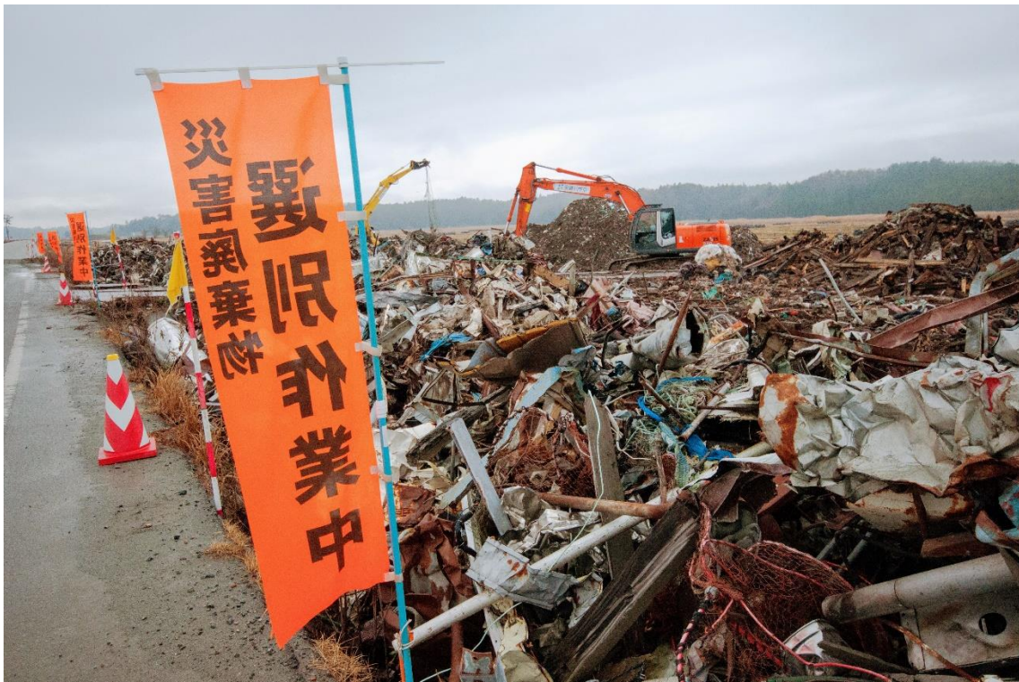
Figure 51: Debris cleanup for coastal zone in Namie begins in 2014 (12/17/2014)
