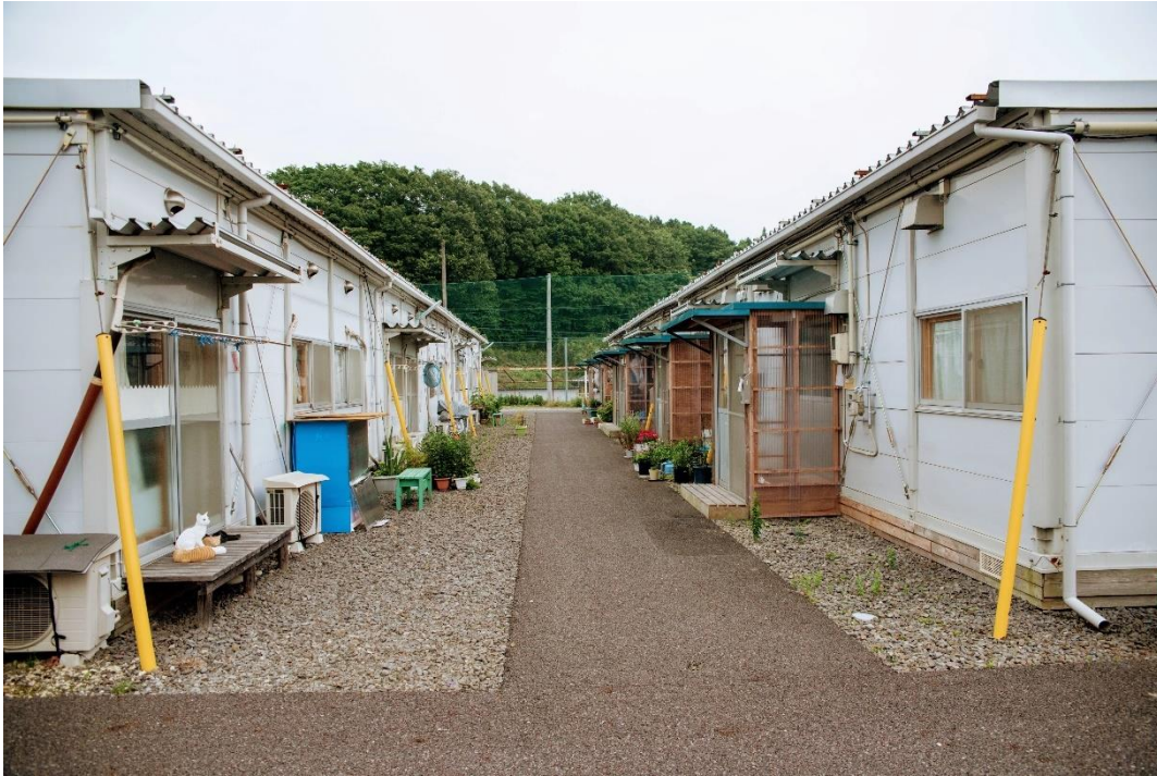
Figure 63: Nihonmatsu evacuation shelter built in a parking lot (7/12/2016)
