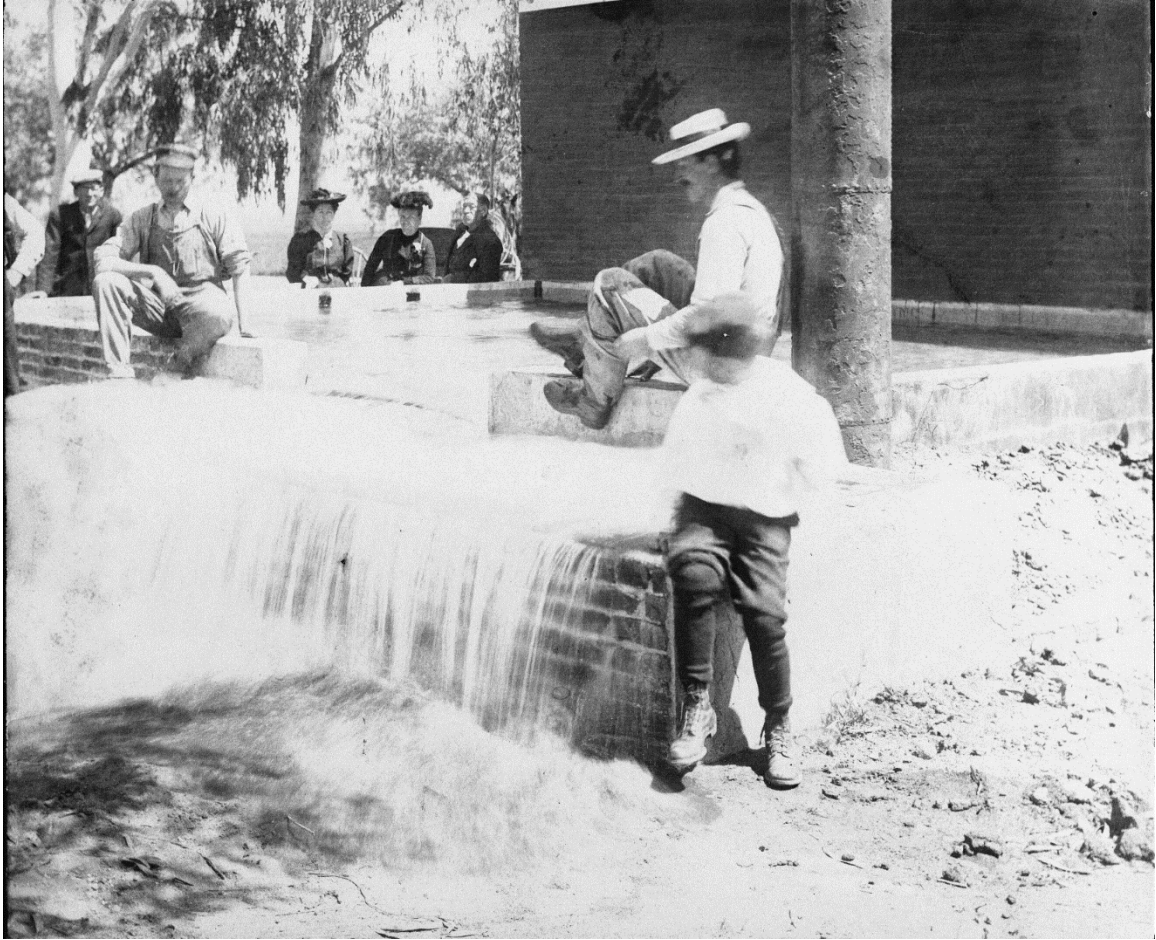
Figure 6. Pumping Plant of Woodward & Sons. William. D. Woodward and his sons G.C. and C.W. had one of the finest alfalfa ranches in east Perris. They built a water pumping plant on San Jacinto Avenue and G Street in Perris. Taken in 1907 this photo shows Mr. Woodward and his family enjoying watching the water flow. His land was irrigated by a 50-horsepower gasoline engine and a No. 8 centrifugal pump. The water was 28 below the ground. They also owned the Woodward Mountain Glen property in Good Hope. (Perris Valley Historical Museum & Association)
