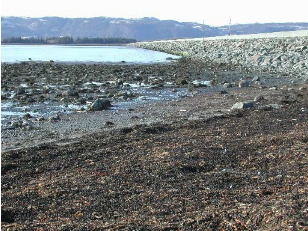
Fig. 5. At low tide, shore areas are exposed on both sides of the embankment, thus allowing animals free passage. This presents a challenge when it comes to finding a wildlife deterrent method that blends in with the natural environment. (Photo: Bjørn Iuell)
