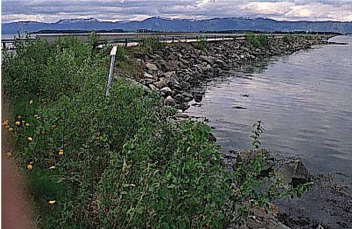
Fig. 4. The embankment emerges as a natural continuation of the shoreline, thus leading animals out to the island. (Photo: Bjørn Iuell)
