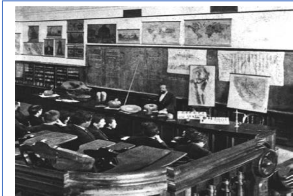
Joseph Le Conte and South Hall Classroom
