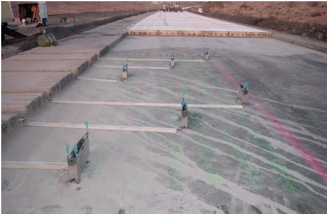
Figure 4. Thermocouples placed in different locations before concrete placement, protected by temporary tin boxes that were removed after placement.
