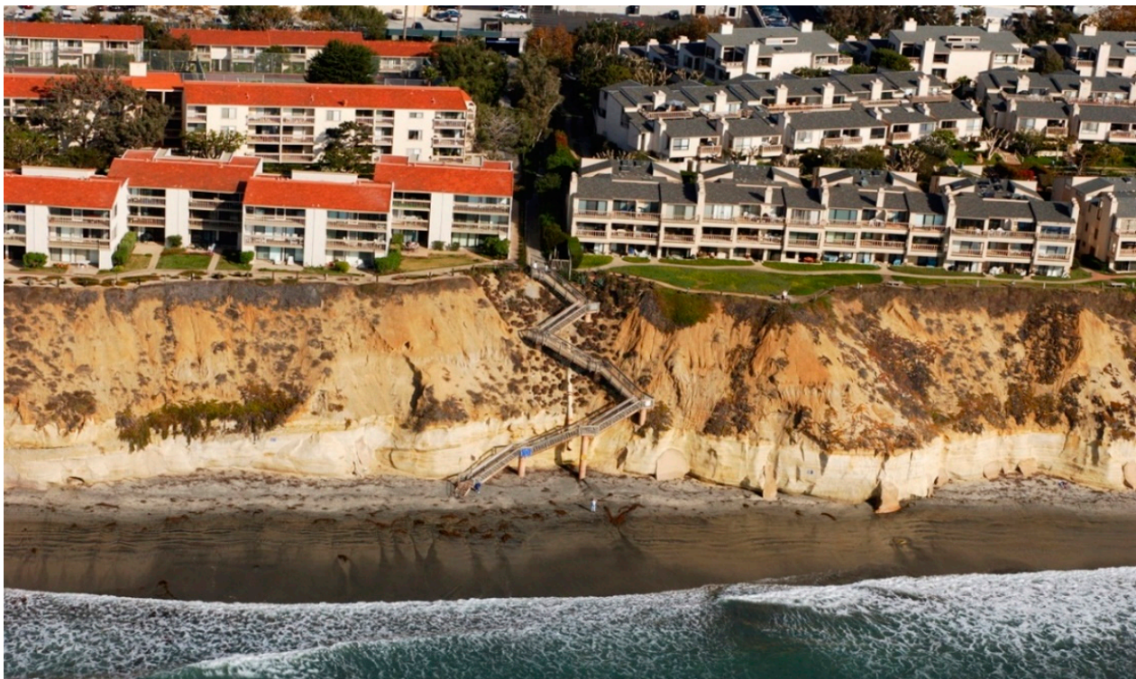
Figure 7. Eroding coastal bluff fronting the lowest marine terrace at Solana Beach, northern San Diego County (Kenneth and Gabrielle Adelman, California Coastal Records Project, Californiacoastline.org ).
