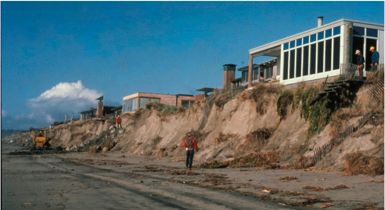
Figure 10. Erosion of a vegetated dune at the Pajaro Dunes development along the central Monterey Bay shoreline during the severe El Niño of January 1983.
