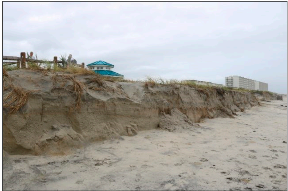
Figure 12. Erosion of vegetated dunes at Sea Isle along the New Jersey coastline during Tropical Storm Ophelia 24 September 2023 (Courtesy of Sea Isle News-Donald Wittowski).
