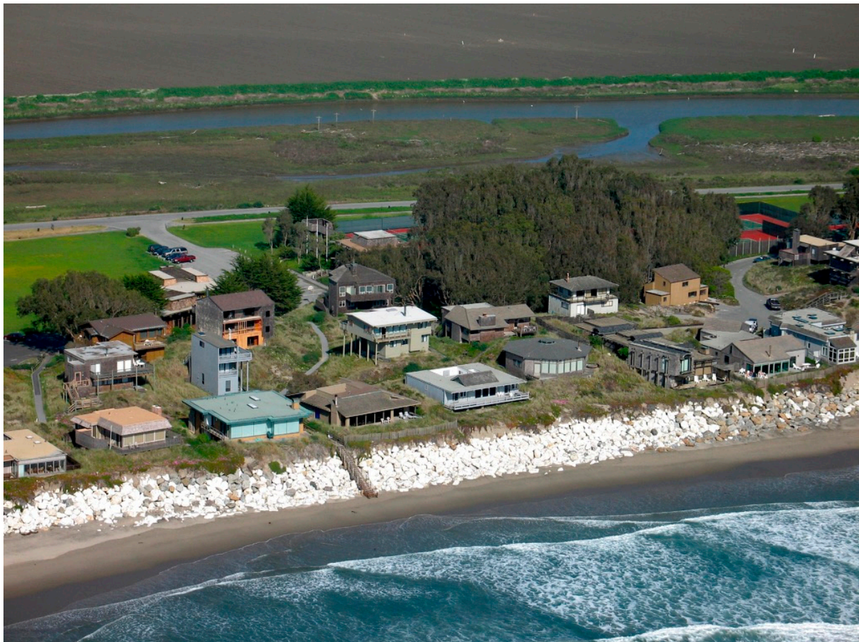
Figure 11. Rip rap revetment placed against eroded dune face at Pajaro Dunes (Photo April 2006).
