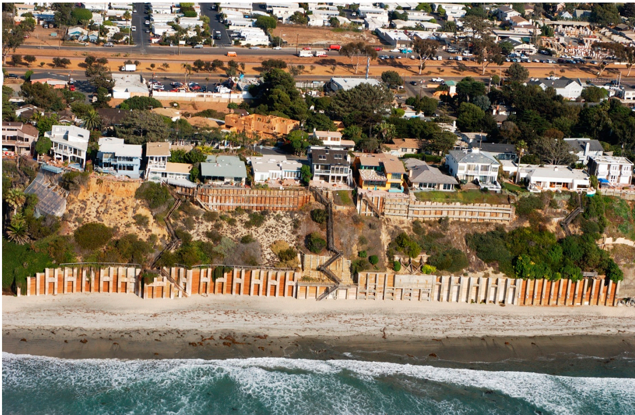
Figure 3. Continuous seawalls along the back beach in Encinitas, northern San Diego County, where 34% of the entire county shoreline has been armored (Kenneth and Gabrielle Adelman, California Coastal Records Project, Californiacoastline.org ).
