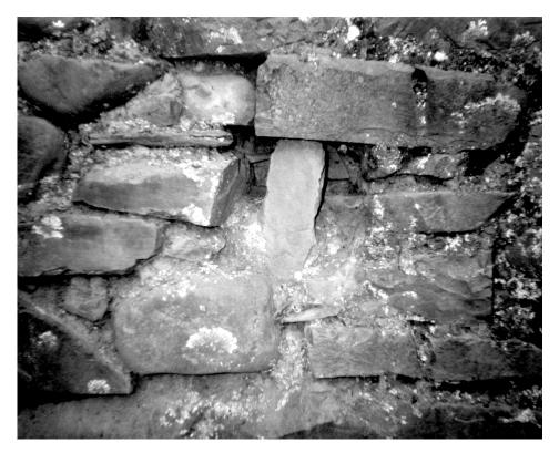
Figure 6.27. Door-bar above the entrance on the interior wall of the east wing.
