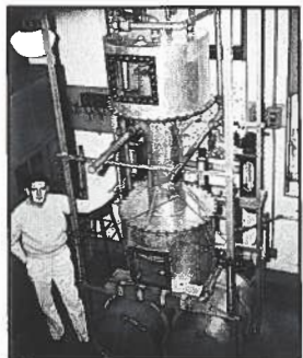
James Crawford, (M.S. '51) with a solvent extraction tower. His research under Wilke led to correlation of limiting flows in extraction towers, which is still the standard today.
