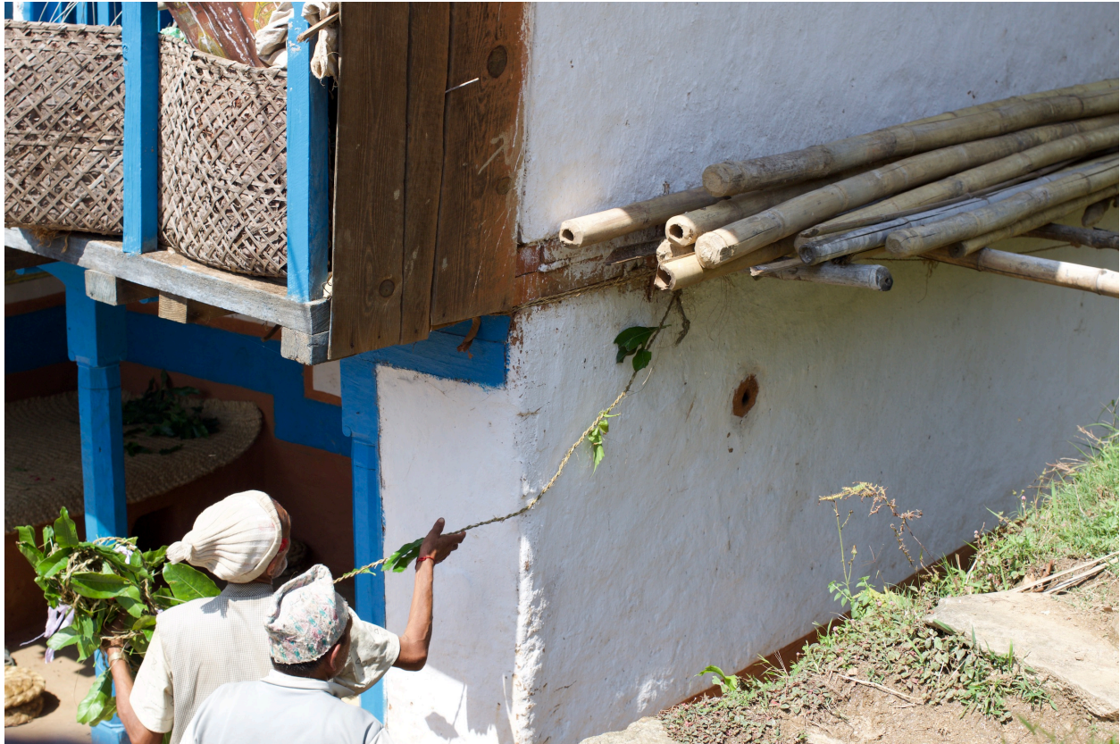
Figure 7 Protecting the house. May 12, 2015.
