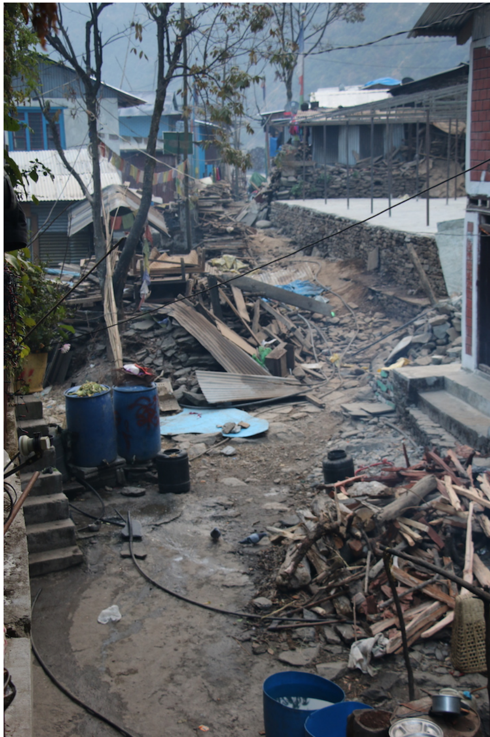
Figure 14 View from our lodgings, eight months after the earthquake. Dolakha.
