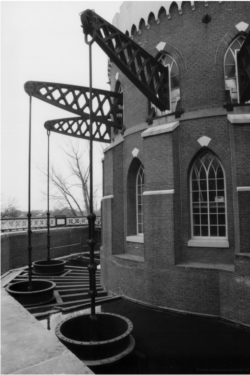
FIGURE 7. Outside view of the Cruquius pumping station. The main cylinder is almost four meters in diameter and is now driven, for demonstration purposes, by hydraulic power. The site has been converted into a museum, and its website ( www.cruquiusmuseum.nl/englishsite/english.html ) gives a full account of the history and mechanics of this engine. Photo by Robert Gisolf.
